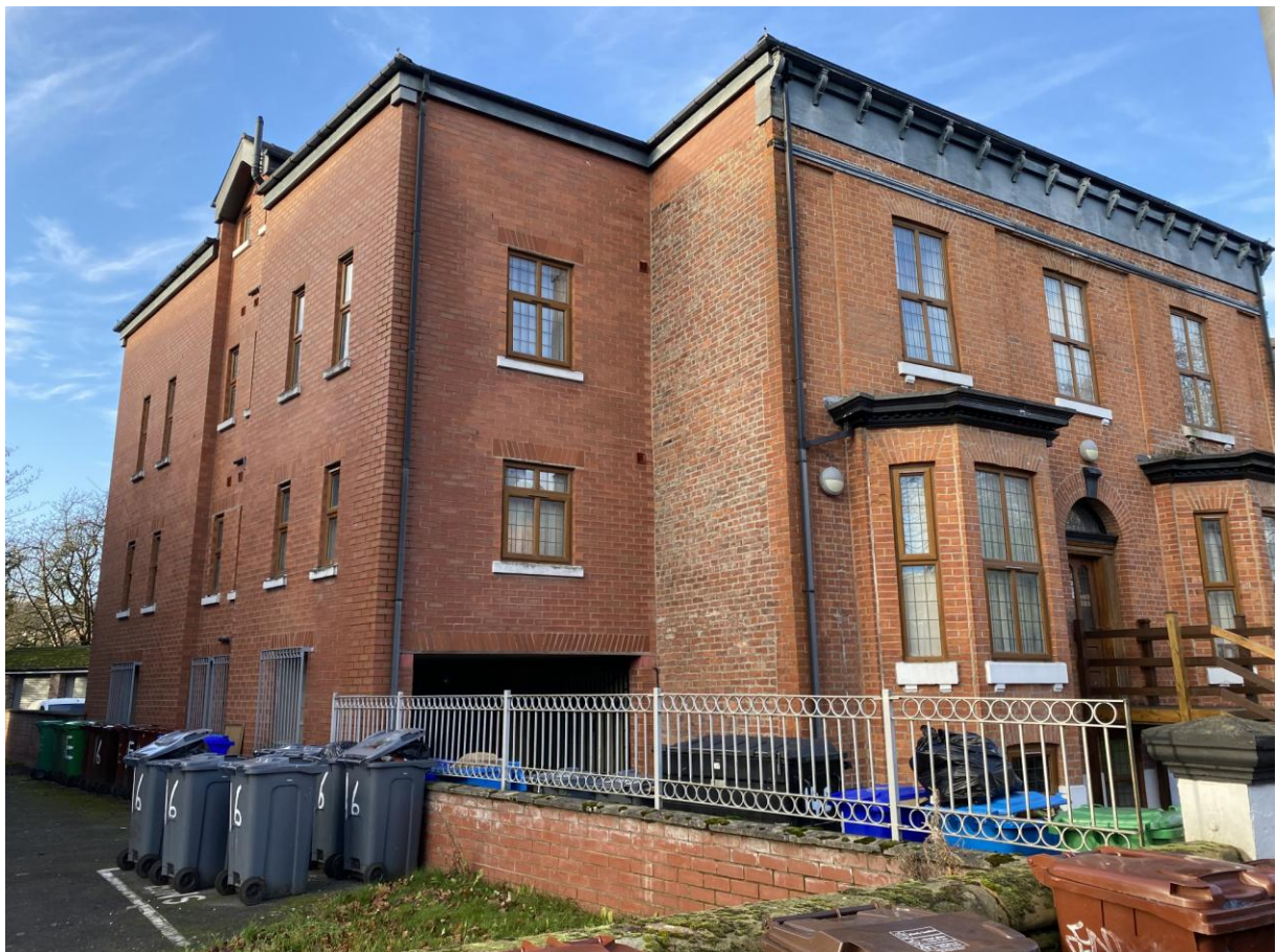
Street View example of neighbouring property 14 Egerton Road, with similar side/ rear projections.
