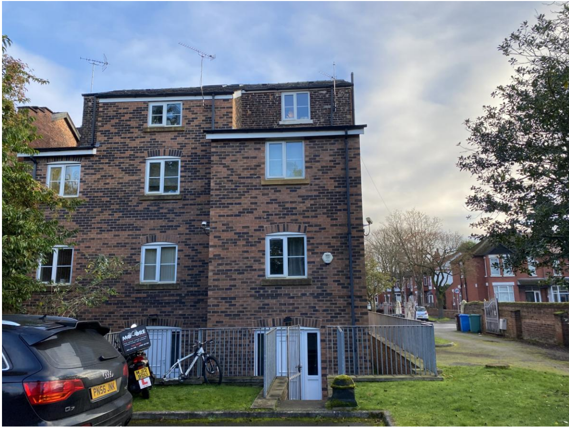
Rear Elevation of existing building.
