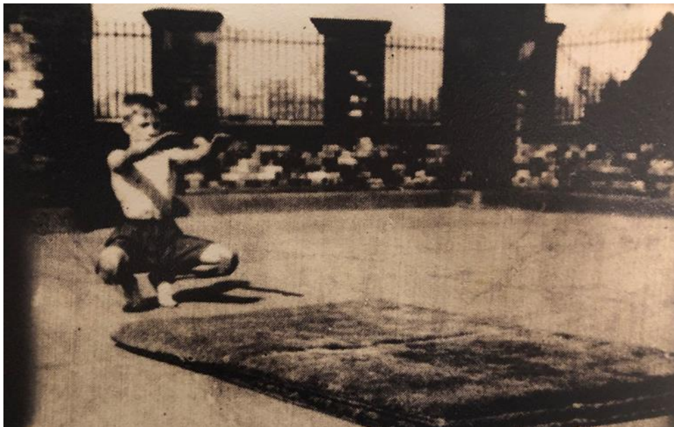
Figure 9: A school boy using the roof top playground for exercise during the 1930s
