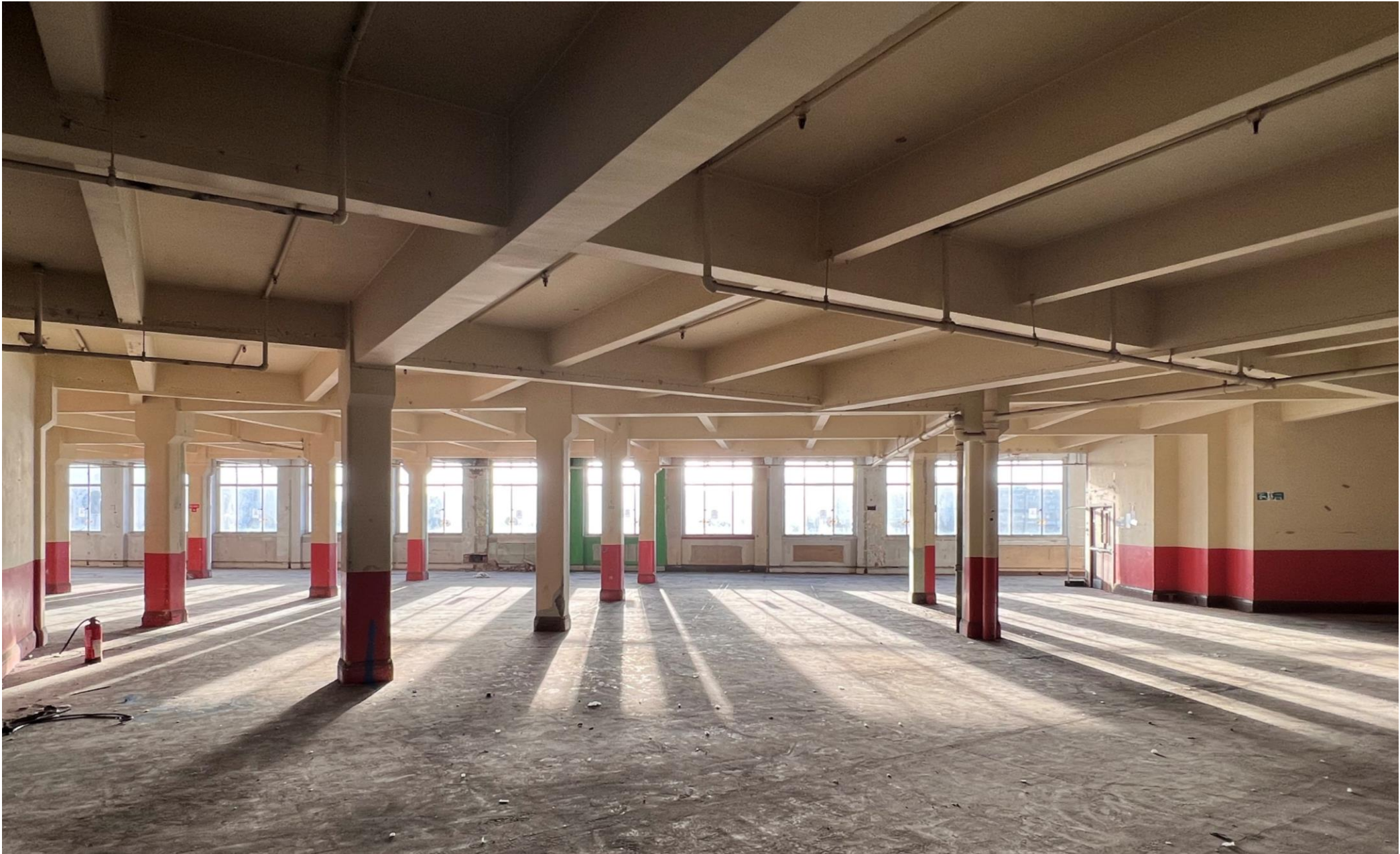
Figure 4 – General view of internal columns.
