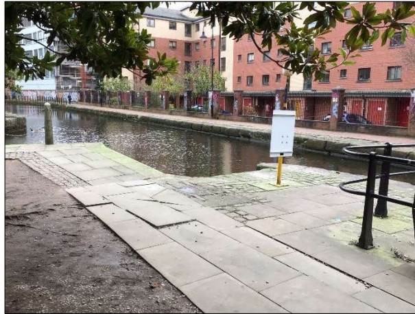
Q14 - Gap between the lock access area railing and post and chain water's edge protection.
