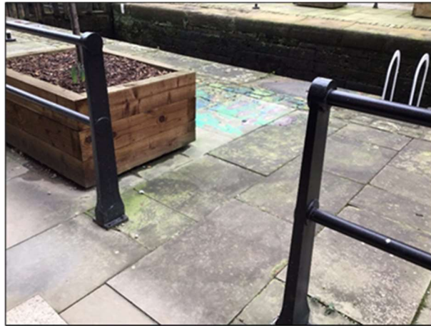
Q11 - Open access point to the lock area.
