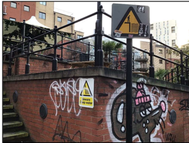
Q2 - Safety signage on the adjacent site was covered in graffiti.
