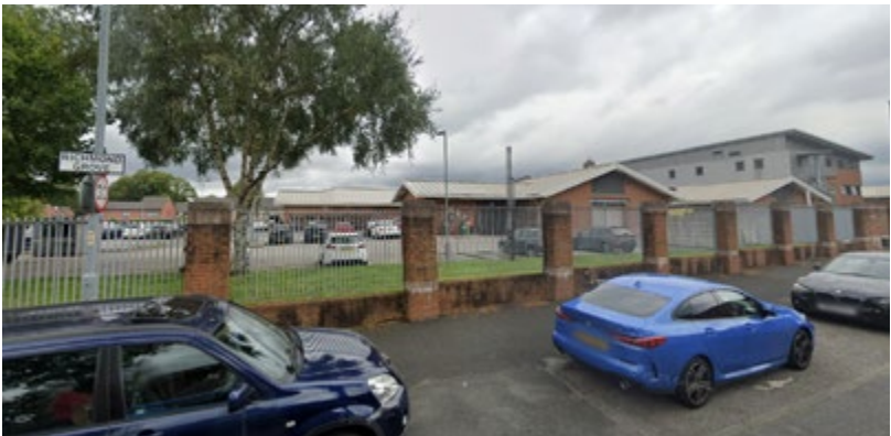
View 01 - From Richmond Grove
