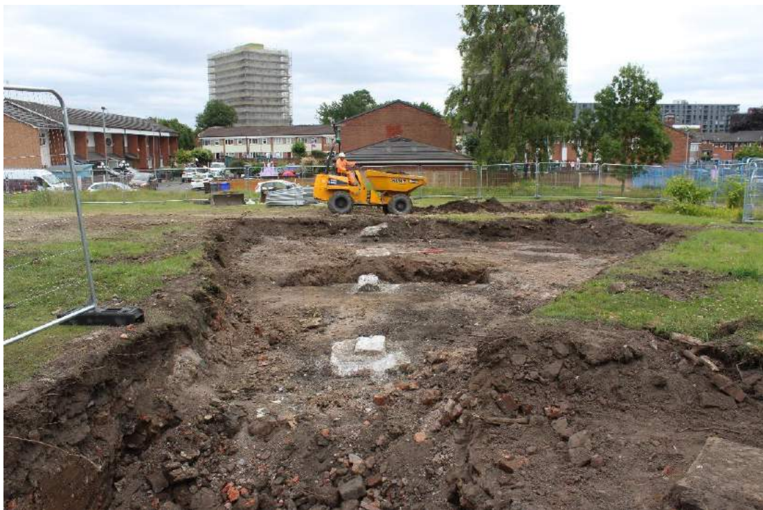
Plate 20: Shot of concrete stanchions {047}, looking south-east. Scale = 1 x 2m.
