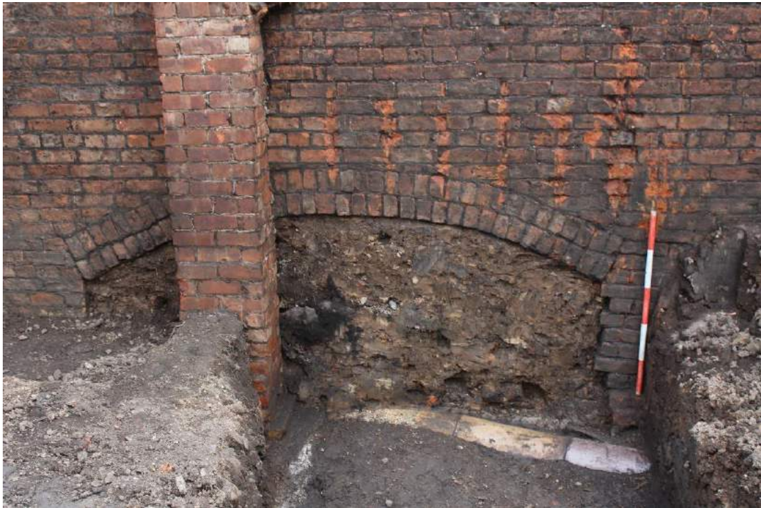
Plate 17: Shot of wall {001} with arch and buttress {006}, looking north. Scale = 1 x 1m.
