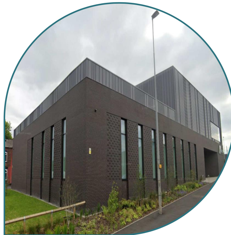
NERIC Building located 3 miles from School
