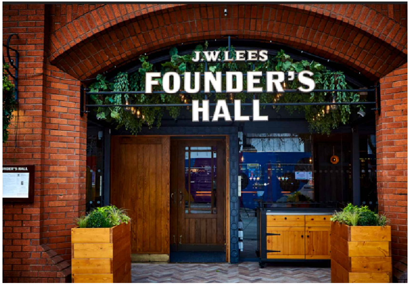
Photograph of as-built main entrance internally illuminated signage and timber pergular ceiling installation
