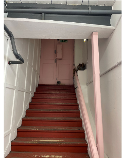
Image 12: Existing Entrance stair
