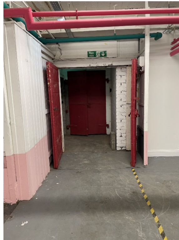
Image 17: Existing Steel exit route doors retained.
