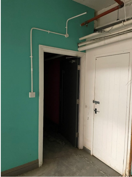
Image 7: Existing Rear stair enclosure. Retained as existing.
