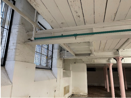
Image 4: Existing ceiling to be overclad.
