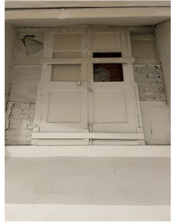
Image 15: Existing high level door retained.
