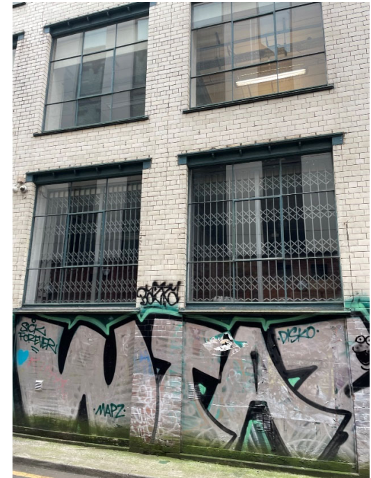
Image 3: Bunsen Street view - End Panel used replaced with new louvre.
