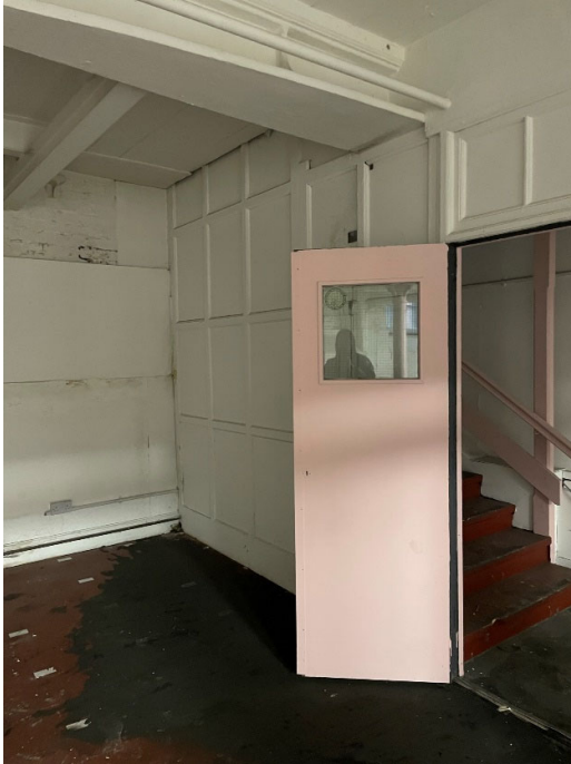
Image 10: Existing entrance to be over boarded.
