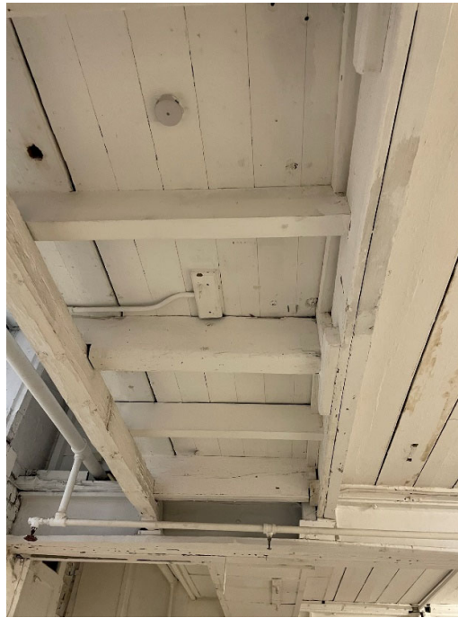
Image 8: Existing ceiling detail to be over clad.
