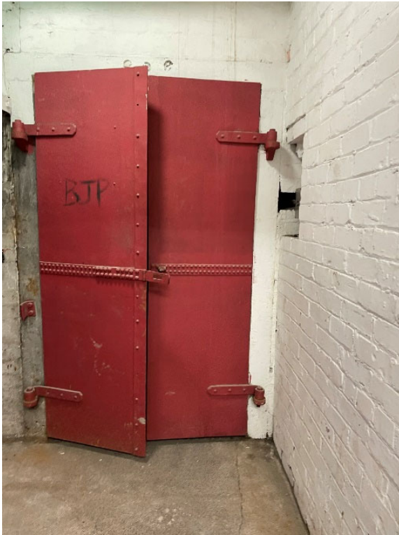
Image 16: Existing Steel doors to lift retained.
