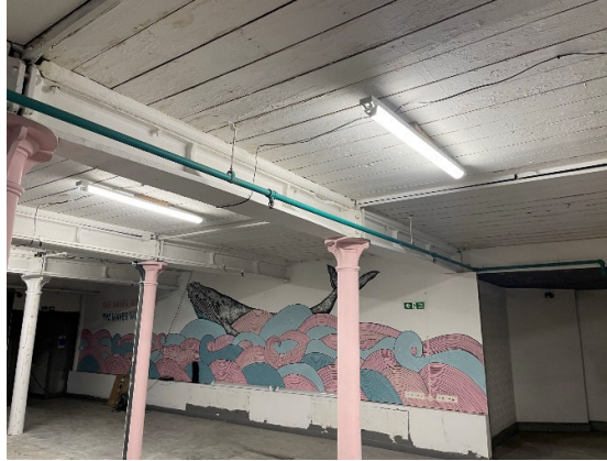
Image 5: Existing photo of existing columns and walls.
