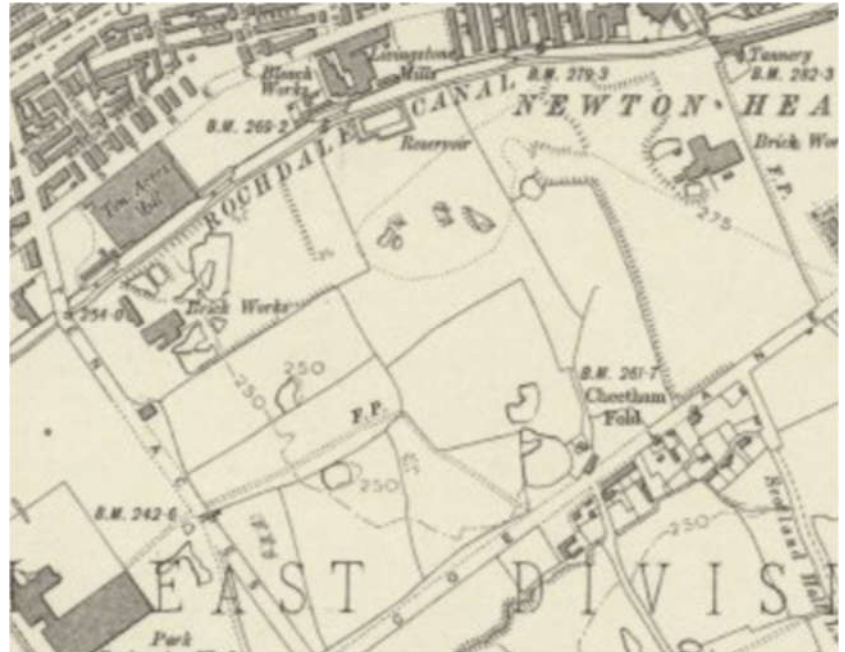
Figure 13 – 1905 – Brickworks constructed to the east and the introduction of outlines of excavations.
