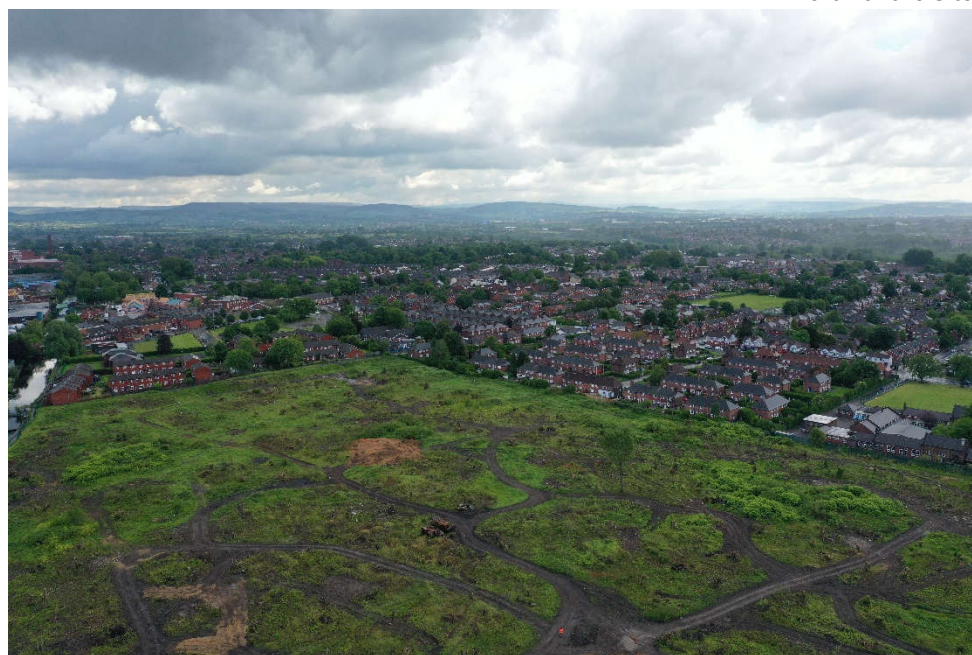
Figure 10-View southeast – views of housing in the immediate area with the primary school to the south of the site to the right of this photo
