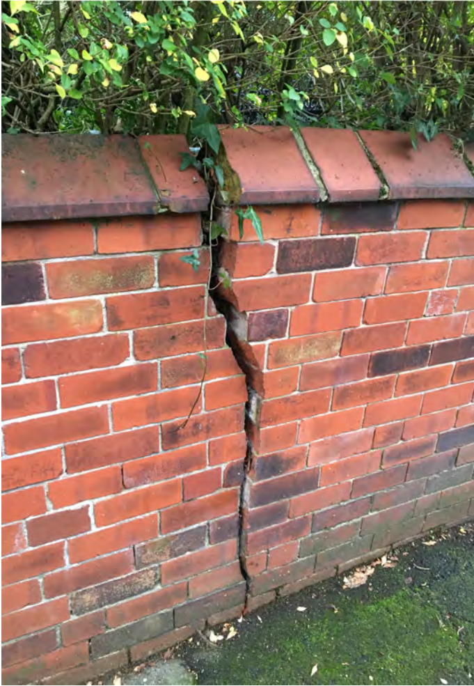
Damage to wall due to T1, T5 & T7
