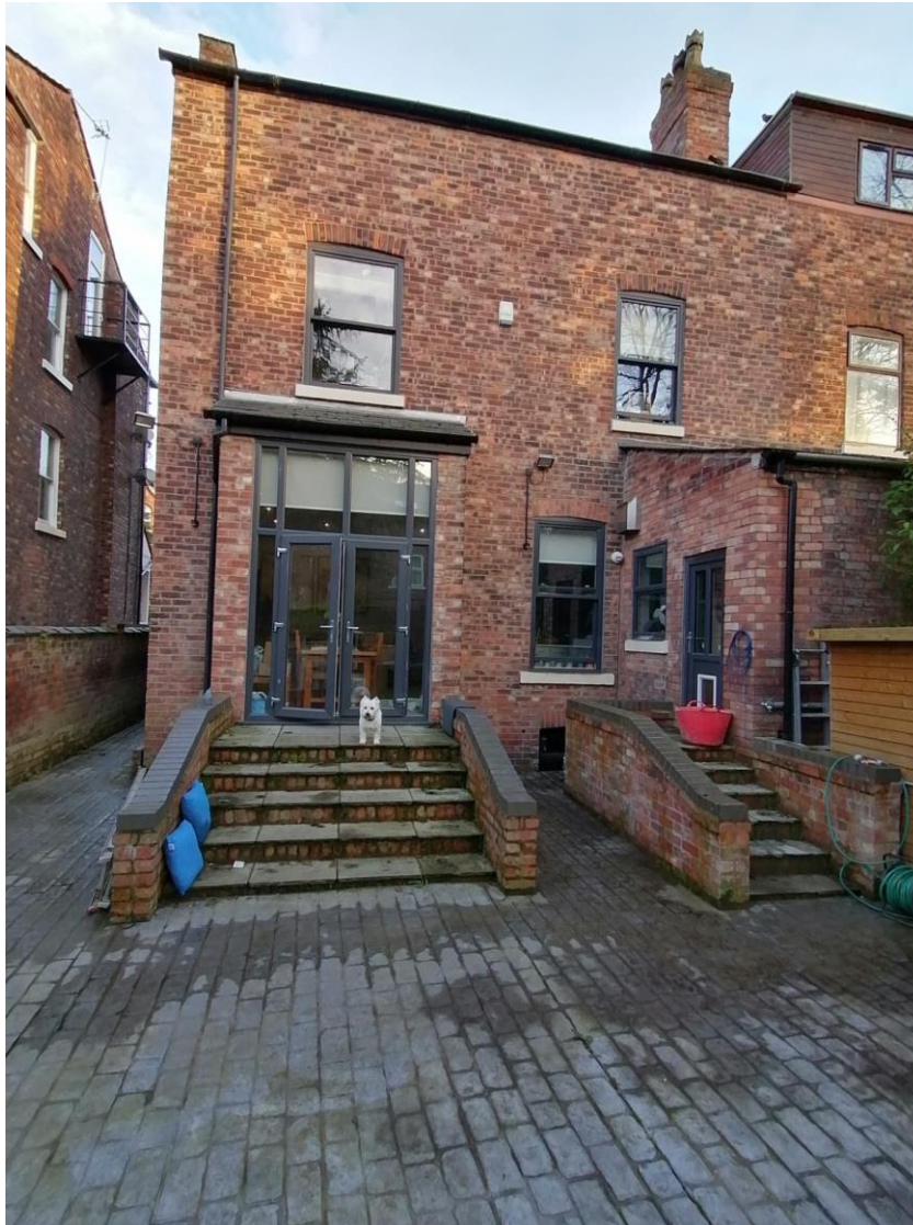
Figure 5: Photograph showing current rear of 100 Clyde Road
