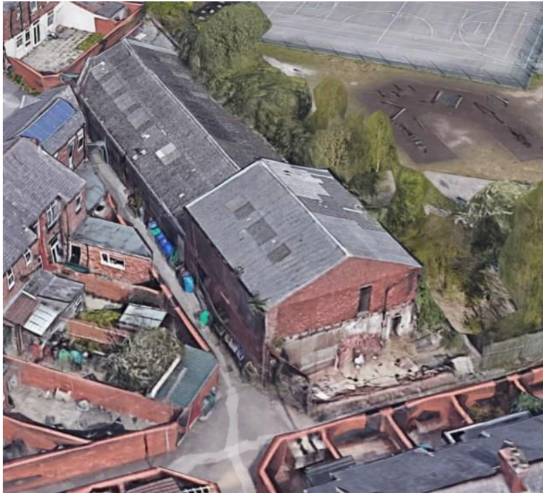
Aerial view of existing building facing north
