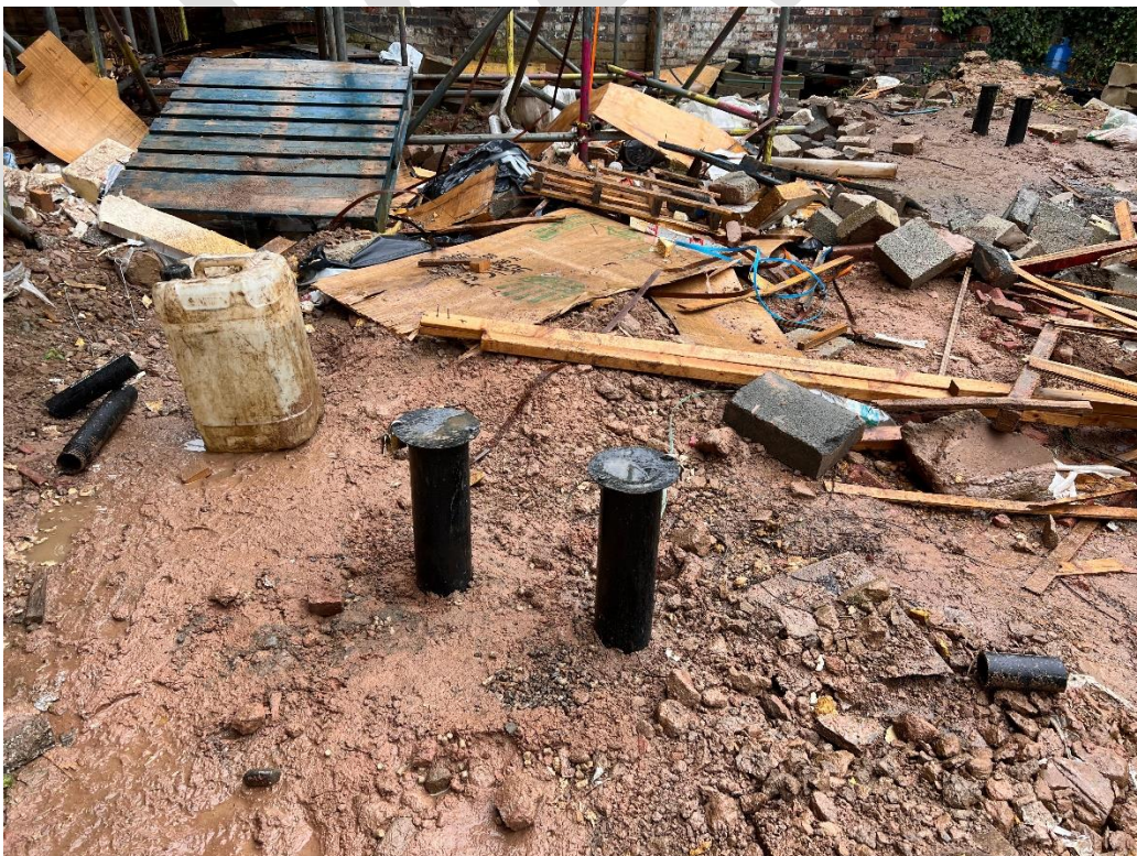
View showing the two monitoring installs, one for shallow 1m vapour installation and a deeper groundwater installation
