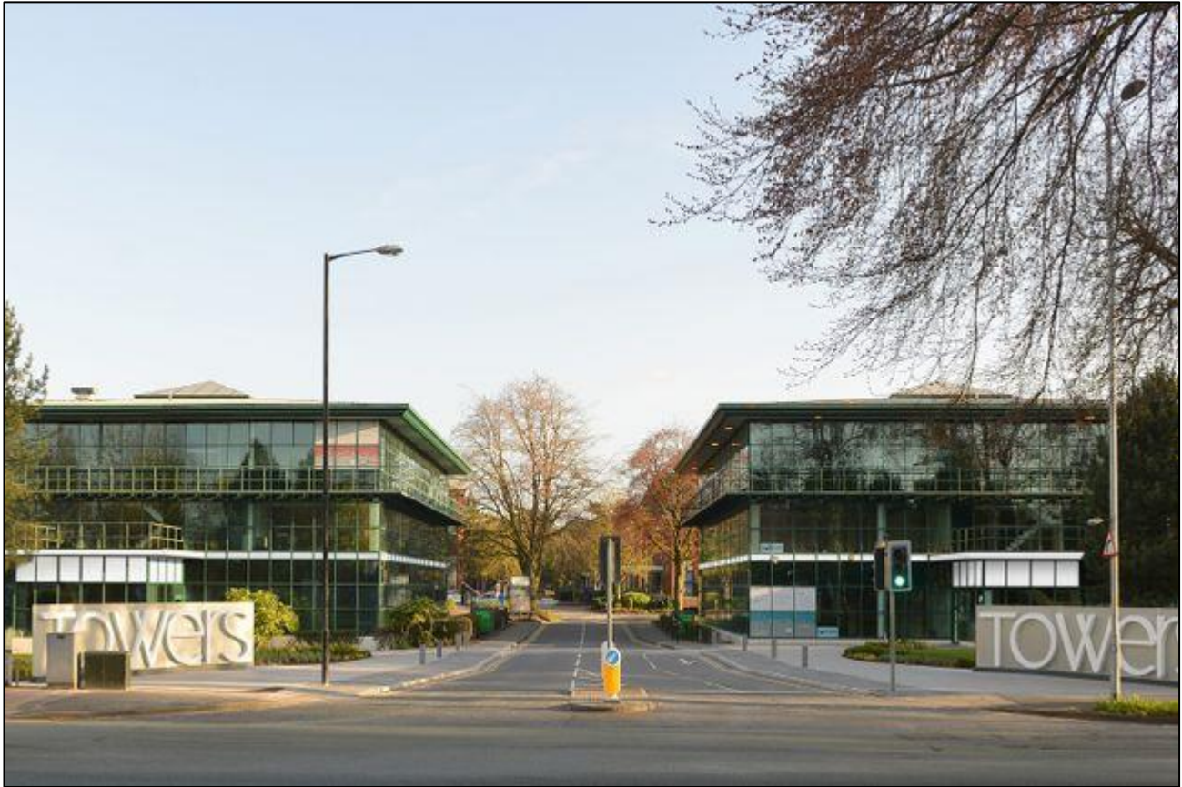
Figure 1. Entrance from Wilmslow Road
