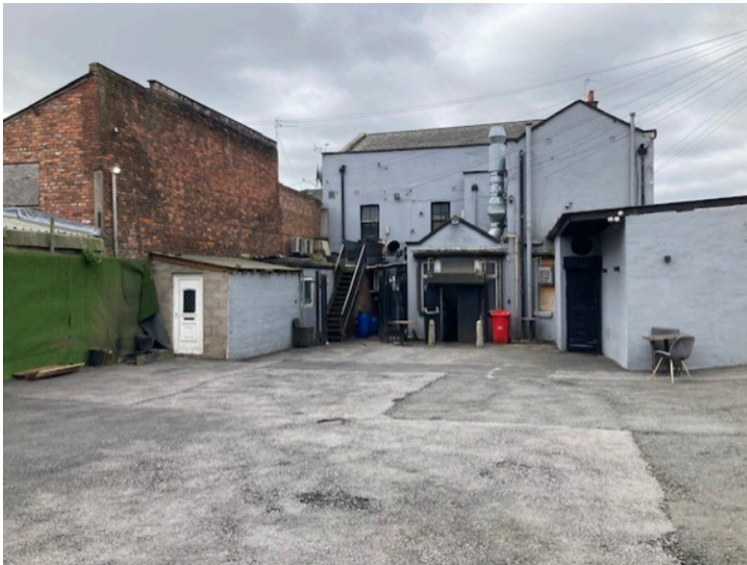
View of rear
