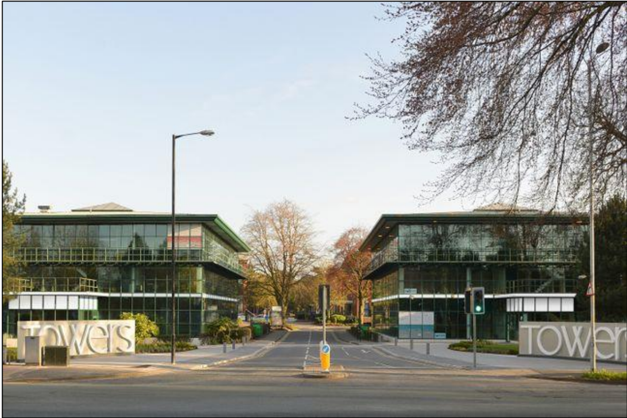
Figure 1. Entrance from Wilmslow Road
