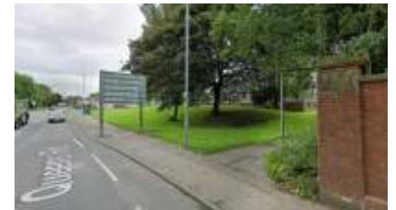
View of Site from Queens Road
