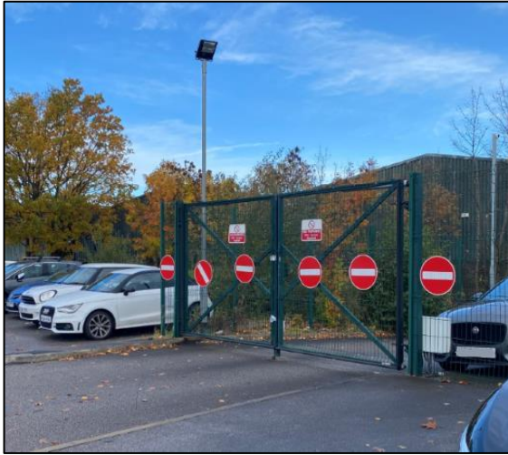
Figure 2.5 (left) – Double Leaf Gate at Staff Car Park Exit
