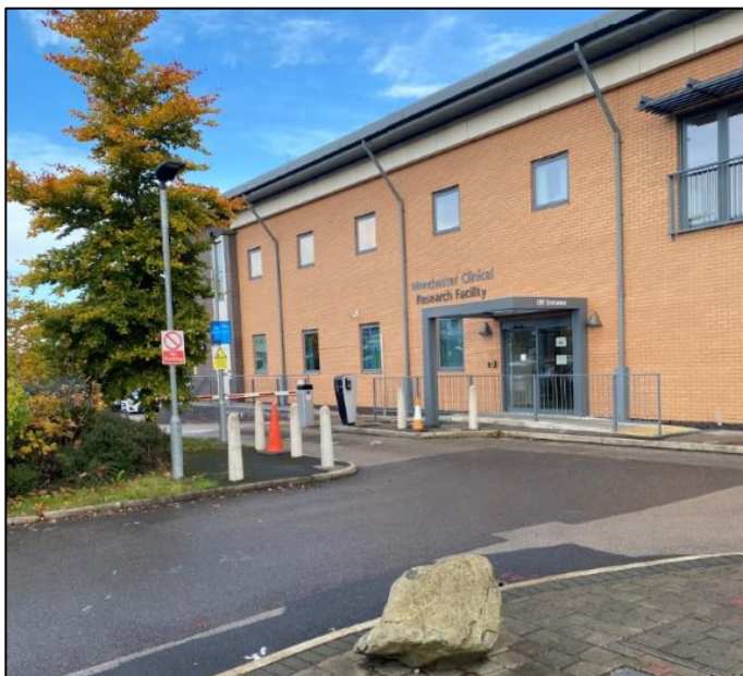
Figure 2.7 – Entrance to CRF Car Park
