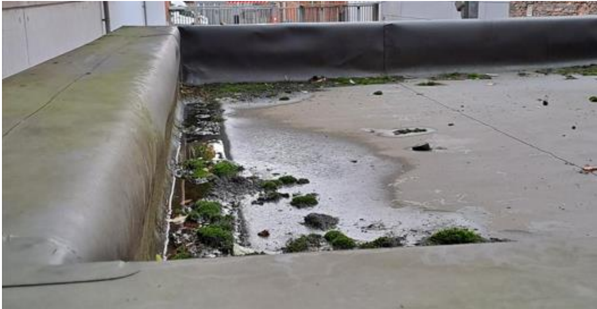
Figure 6. Flat bitumen roof of security building.
