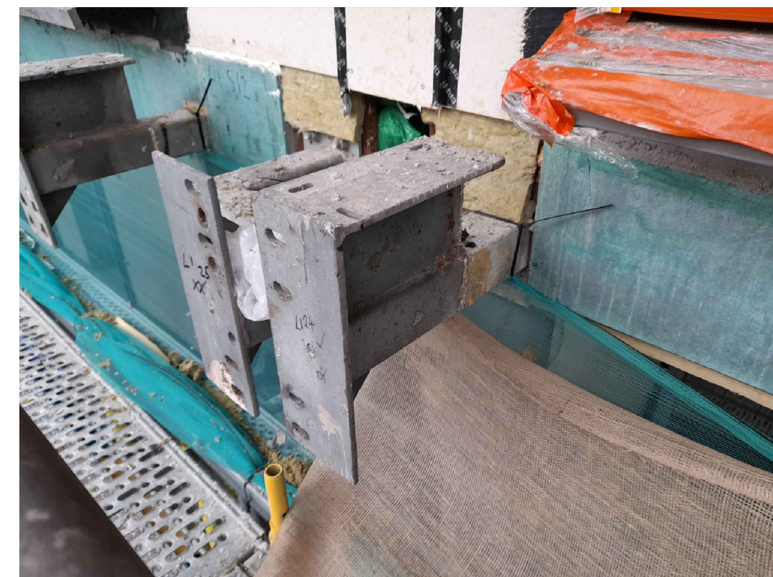
PHOTOGRAPH SHOWING FACE OF WALL TO GINNEL 1ST FLOOR
