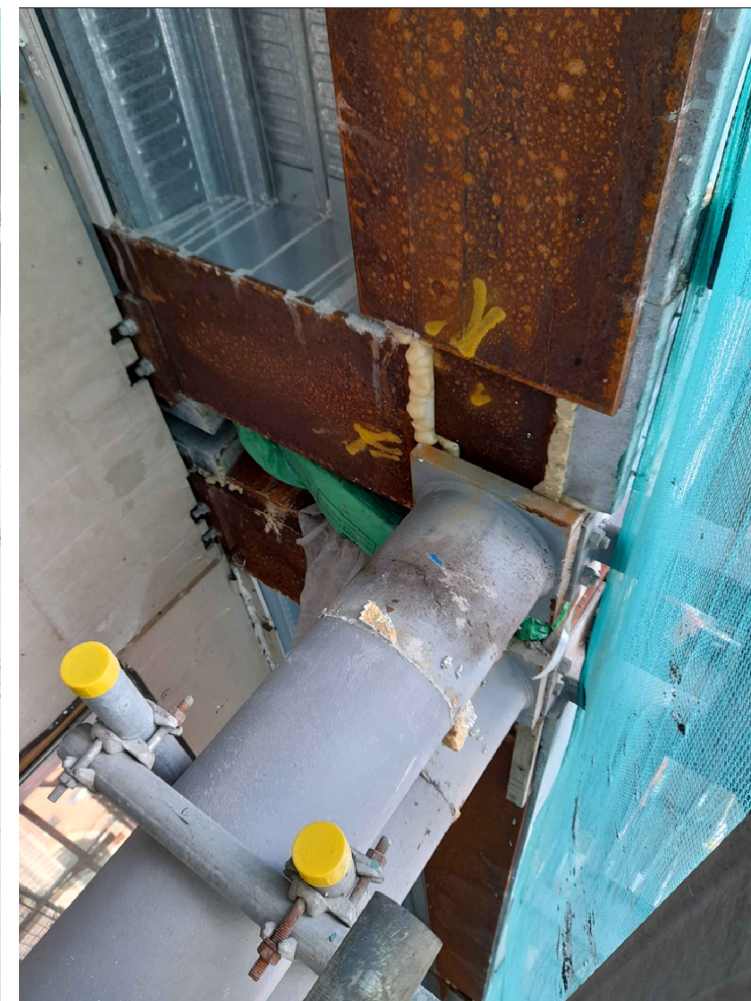
PHOTOGRAPH SHOWING U/S OF SOFFIT TWO COLUMNS TO GINNEL
