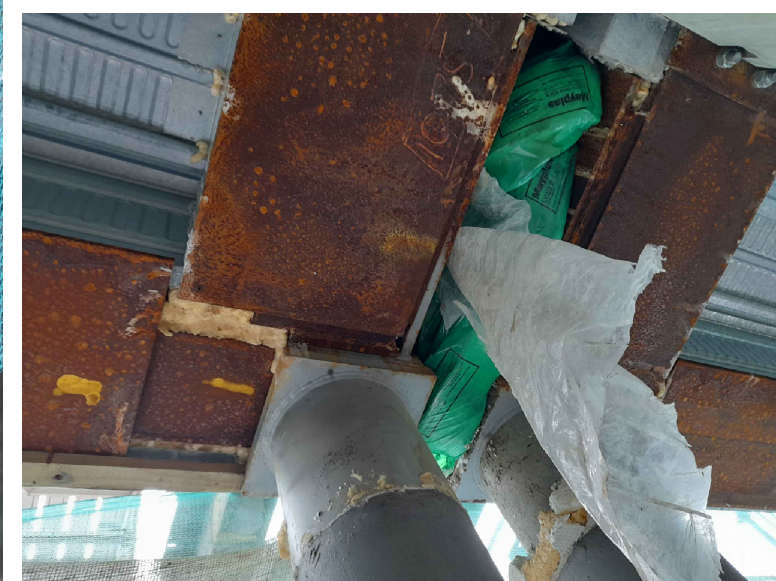
PHOTOGRAPH SHOWING U/S OF COMBIDECK SLAB TO GINNEL
