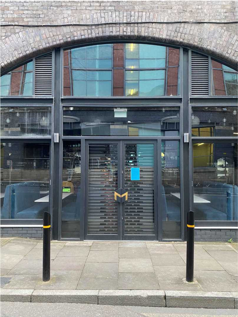
No 10 -15 ALL WINDOWS TO BE ALUMINIUM PPC TO MATCH FRAMES OF PLANNING REF: 122070/FO/2018. DARK GREY
