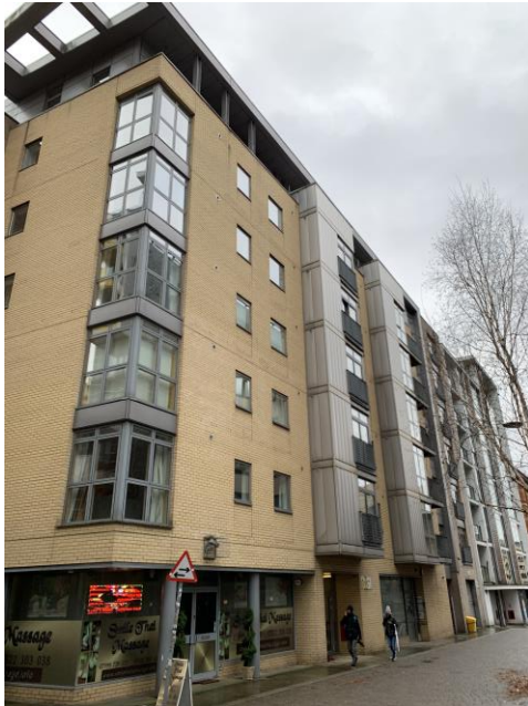
Figure 2.2: View of the application building (west elevation).
