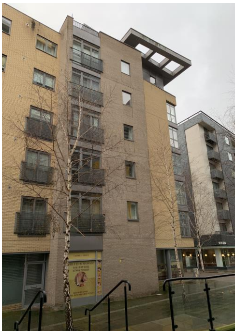
Figure 2.3: View of Garden House (north elevation).
