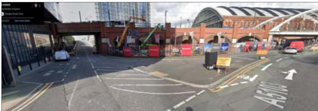
Figure 3.1: Albion Street/ Trafford Street Junction
