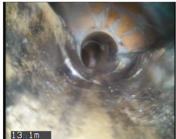
MH4X_c72011d5-567b-42df-b57e-b0b97a1b682b_20230706_162504_568.jpg, 00:01:25, 13.20 m Finish node, manhole, reference: Discharge, MH5 (Buried)
