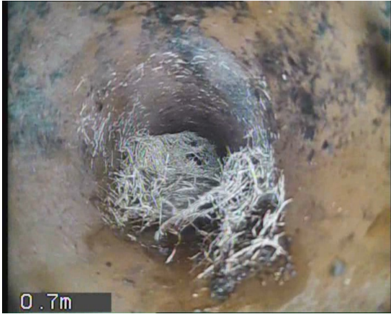
HOLX_8b7d95bc-b8ef-4f2a-9f80-63491000b28e_20230706_1 45747_645.jpg, 00:00:11, 0.80 m Roots, mass, 100% cross-sectional area loss
