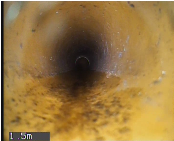
HOLX_4ab13148-c682-4458-936e-7e84e96c06df_20230706_141351_920.jpg, 00:00:44, 1.50 m Pipe material changes to polyvinyl chloride at this point
