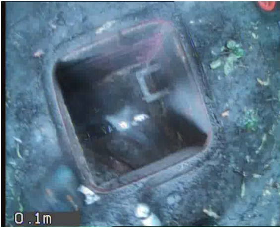
HOLX_bf044e95-4274-443b-a248-26ec7f06f272_20230706_144542_575.jpg, 00:00:00, 0.00 m Start node, manhole, reference: MH1 B1
