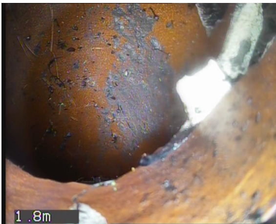
HOLX_9afadac9-e2fa-45be-98cb-f03a69889fb9_20230706_1 64450_725.jpg, 00:00:26, 0.00 m Joint displaced, large
