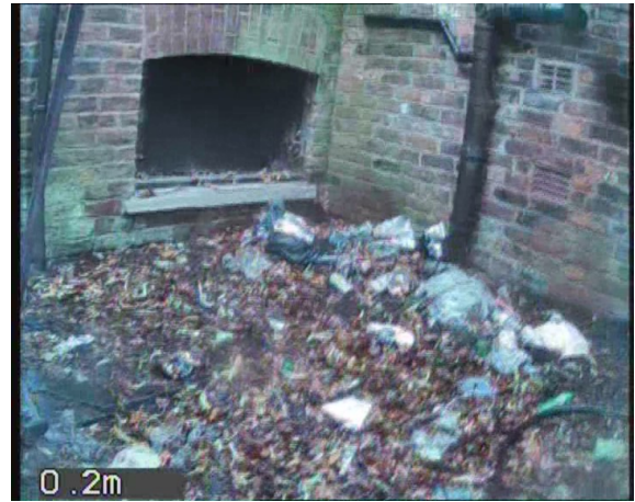
HOLX_1e49bc03-7cb6-40a1-949b-1ed1152b80c2_20230706_144547_861.jpg, 00:00:00, 0.00 m Start node, manhole, reference: MH1 B1
