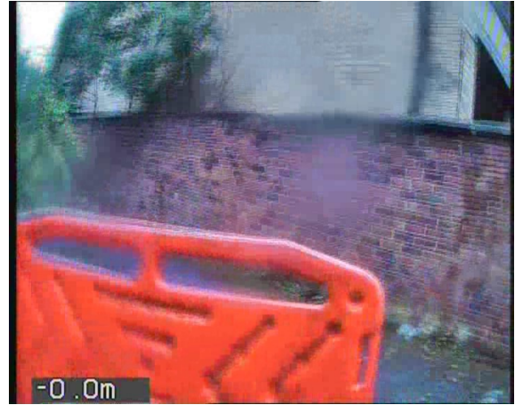
HOLX_d0f274f8-9c2d-4a60-8e2f-77648aa782c0_20230706_1 64248_620.jpg, 00:00:00, 0.00 m Start node, manhole, reference: MH3
