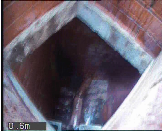
MH2X_e57c65de-4a54-4ee1-83c5-3c710a1092ae_20230706_150852_096.jpg, 00:00:00, 0.00 m Start node, manhole, reference: MH2
