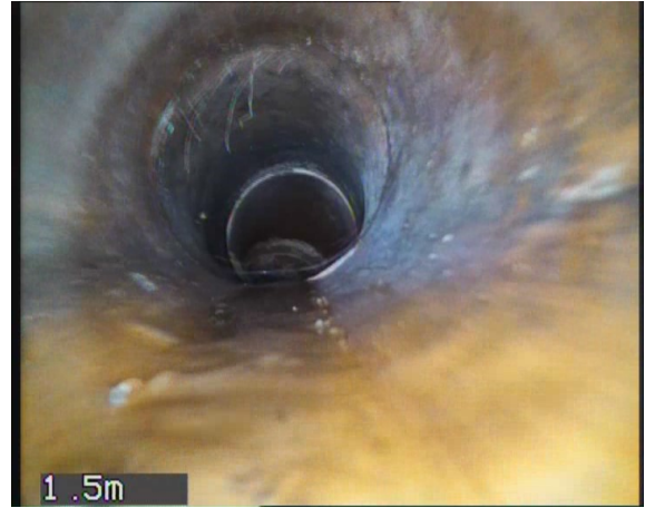
MH2X_e63b2c25-b512-474a-b5dc-6a9fbf5f667d_20230706_151040_723.jpg, 00:00:50, 1.60 m Roots, fine
