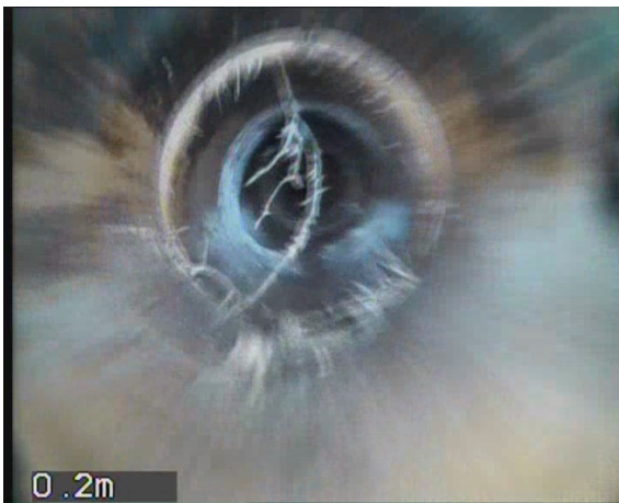
HOLX_f19a829c-729a-4d22-b119-50254150705c_20230706_144741_205.jpg, 00:00:36, 0.30 m Roots, fine at joint
