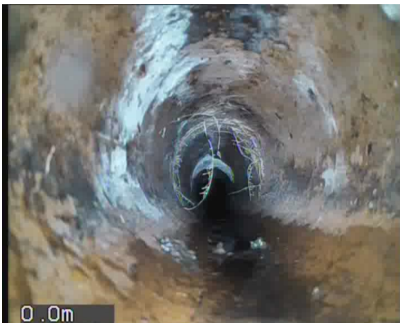
HOLX_296dc49c-b433-46e6-b823-476ff07f555d_20230706_141149_423.jpg, 00:00:28, 0.50 m Roots, fine at joint
