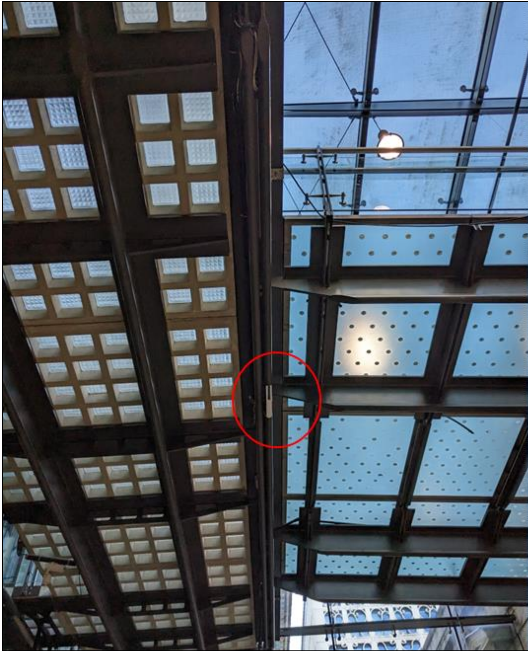
Appendix 18: GFAP6 situated in GF002 Atrium is to replace the existing access point (highlighted in the above photograph) like for like. GFAP6 is to be fixed to the ceiling using a steel bracket, mirroring existing fixtures in the Atrium. As such the changes to the buildings fabric and character are negligible.
