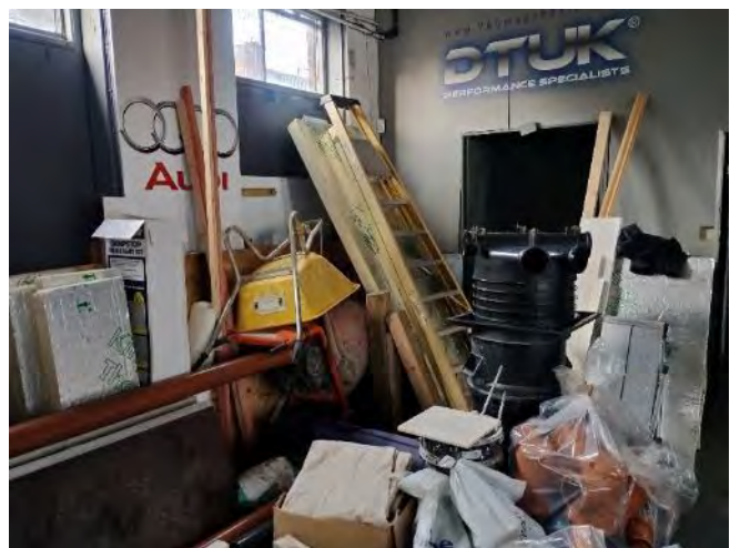
Figure 24 – Debris build up in the southern section of the garage including a ladder, plastic pipes, sheets of foam, wooden panels and cardboard boxes.
