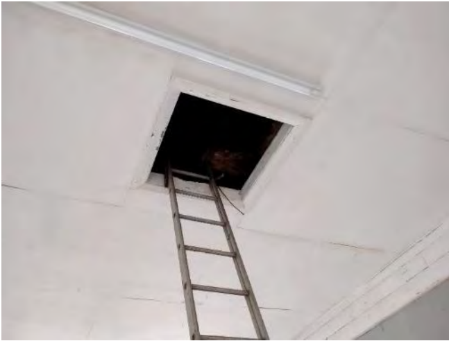
Figure 31 – Access into the loft area of the garage building in the southern site section.
