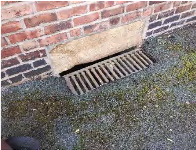
Figure 21 – The grate leading into the sump from ground level.
