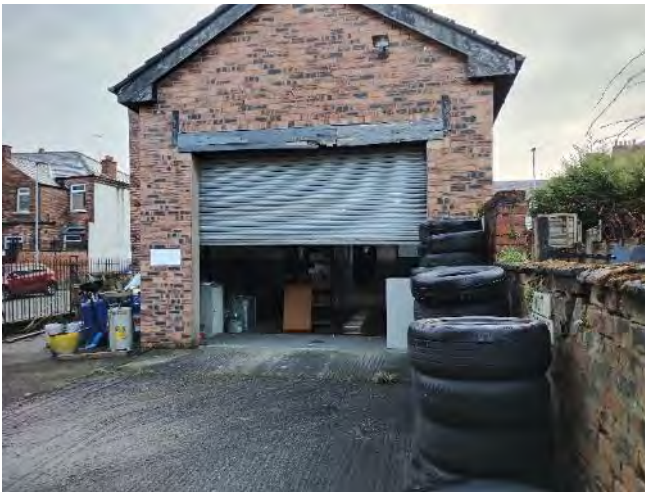
Figure 3 – Entrance to the garage from the northern site section
