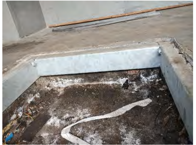
Figure 10 – Beneath the pits appear to be lined with concrete and bricks
