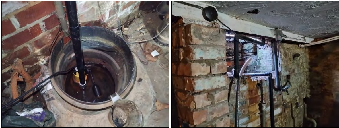
Figure 5: Photographs showing the sump in the basement leading to a grate on ground level
