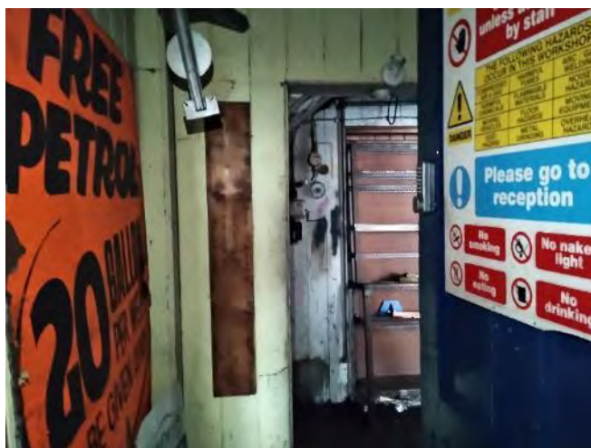
Figure 27 – Access into the garage from the southern site entrance
