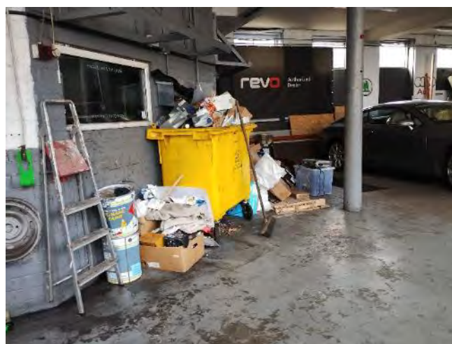
Figure 30 – Waste in the southern section of the garage including paper, a ladder, weathered paint tins and plastic packaging.
