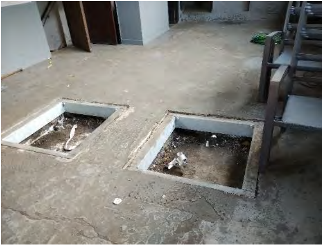
Figure 9 – Two sunken pits in the floor in the centre of the garage.
