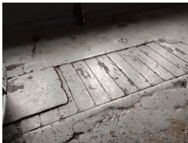
Figure 28 – A boarded up pit in the southern section of the garage.
