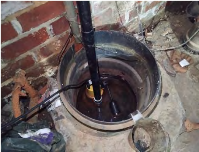
Figure 19 – The sump located in the basement.
