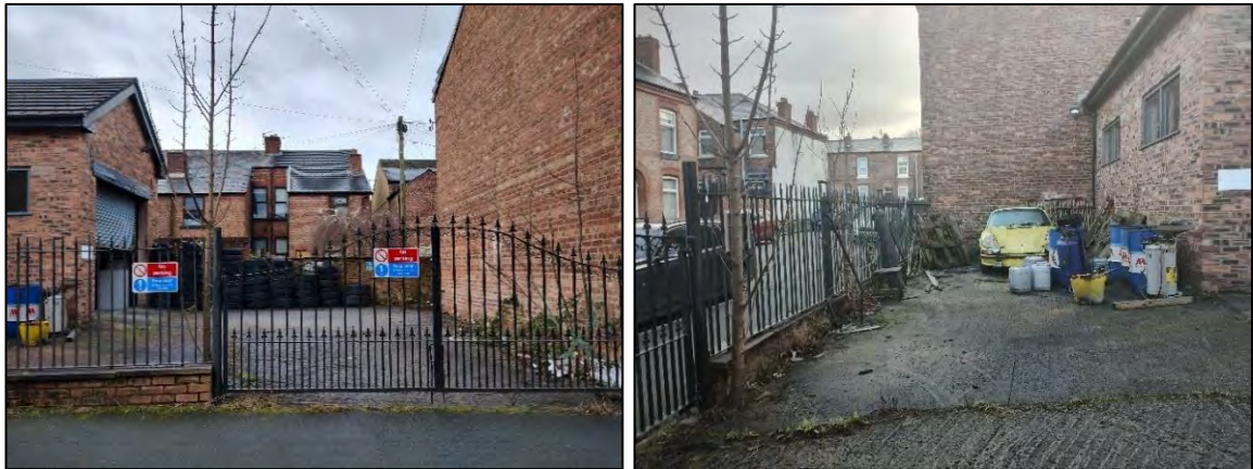
Figure 4: Photographs of the yard in the northern section of the site.
