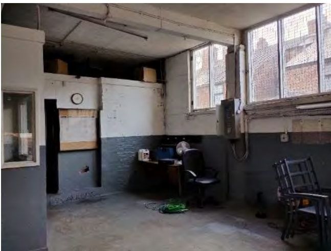
Figure 11 – The centre of the garage area
