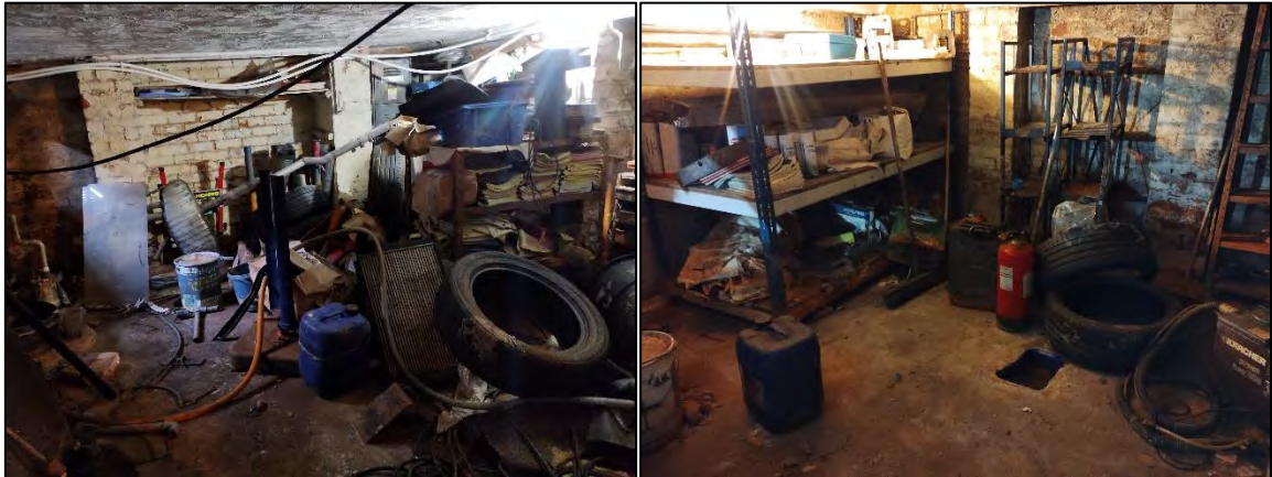
Figure 7: Photographs showing the debris in the basement.
