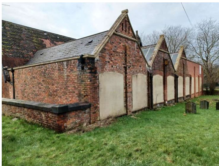
1. Photo of north elevation taken from Church of Cross grounds
