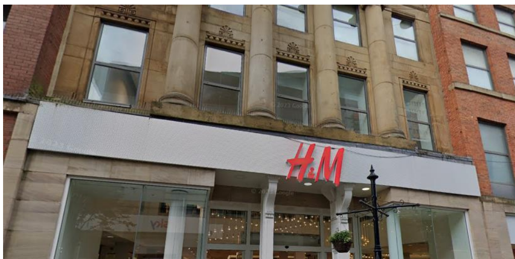
Figure 1: Former Fascia (c.2012 – July 2023)
