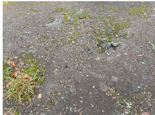
Photograph 10: Melted plastic present on the informal footpath surface, east of Dam Head Drive.
