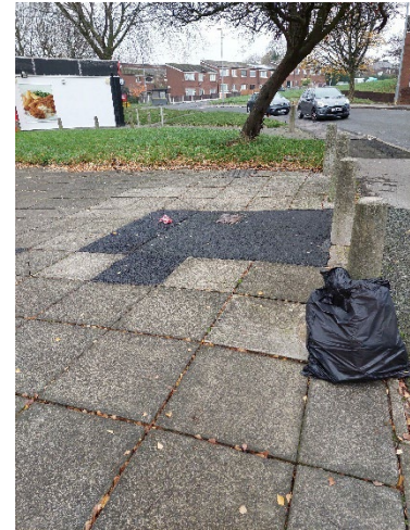
Photograph 20: Bag of rubbish outside One Stop Convenience Store off Haverfield Road.
