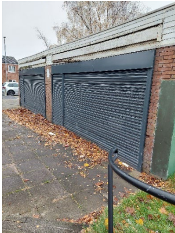
Photograph 19: Unoccupied shopping units next to the One Stop Convenience Store, south of the site.
