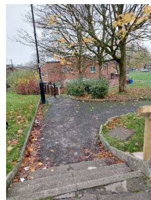
Photograph 18: Narrow passageways to the rear of the Convenience Store.
