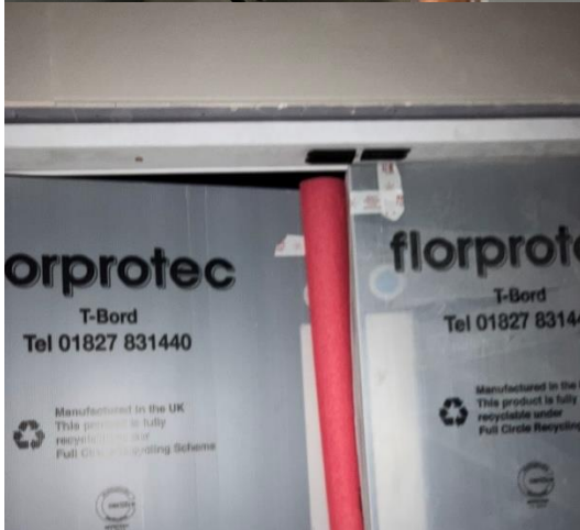
Figure 2 Un-closable Record Room doors
