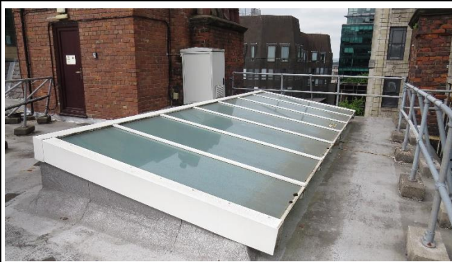
Upper Roof with Lantern and Lift Shaft Housing
