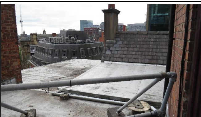
Southwest Corner of Upper Roof
