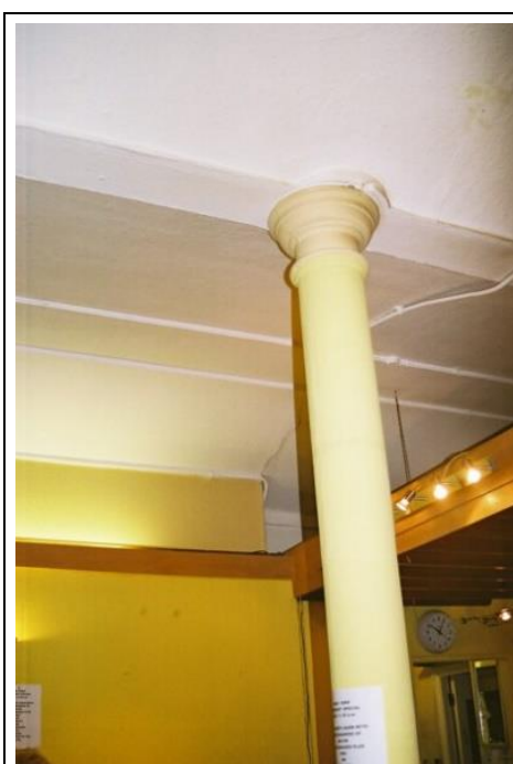
Cast Iron Pillar and Brick Jack-arch
