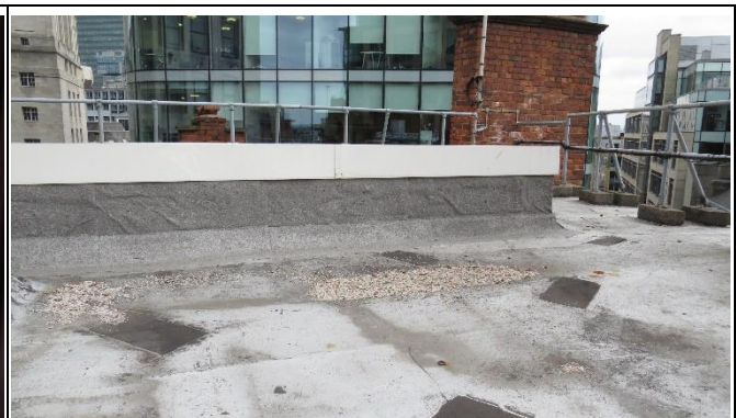
Central Area of Upper Roof
