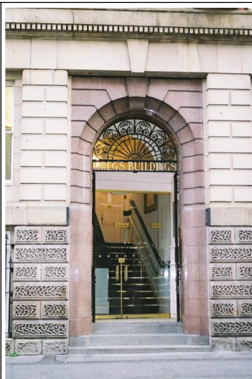
Main Entrance, Booth St. Elevation
