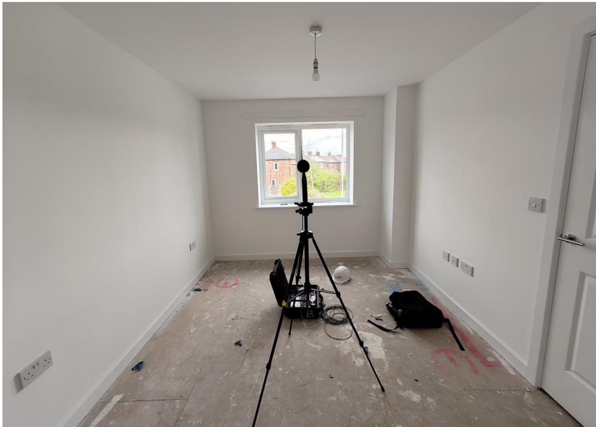
Figure C4: Site Photographs – Plot 11 / Block 6 Front Bedroom
