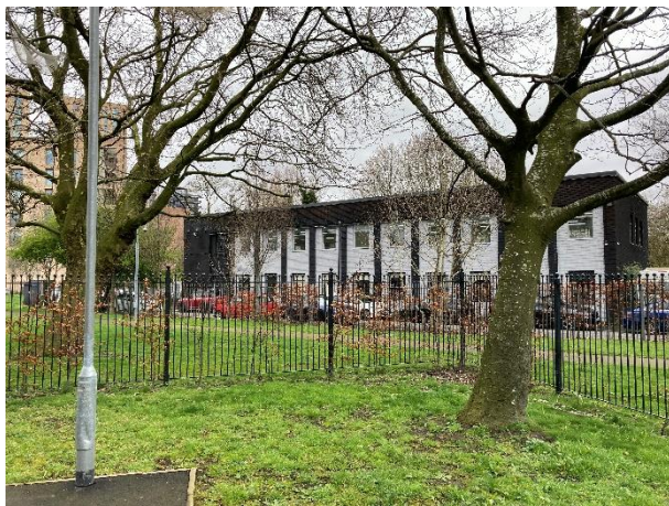
3.15: View of front elevation of Palmer House (fronting Virgil Street)
