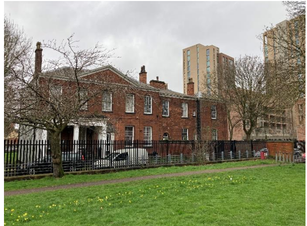
3.20: View of front elevation of Hulme Barracks and adjoining Botanica development.
