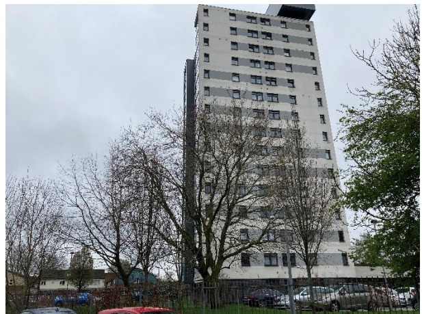
3.16: View of Princes Court Tower building.
