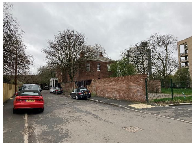
3.18: View of the side elevation of Hulme Barracks.
