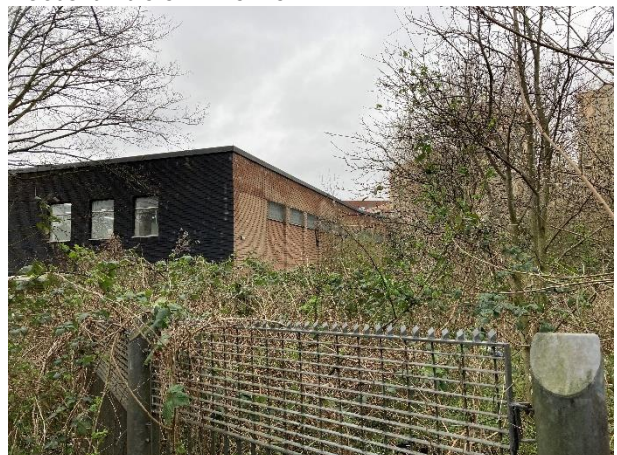
3.12: View of rear elevation of Palmer House and currently inaccessible land.
