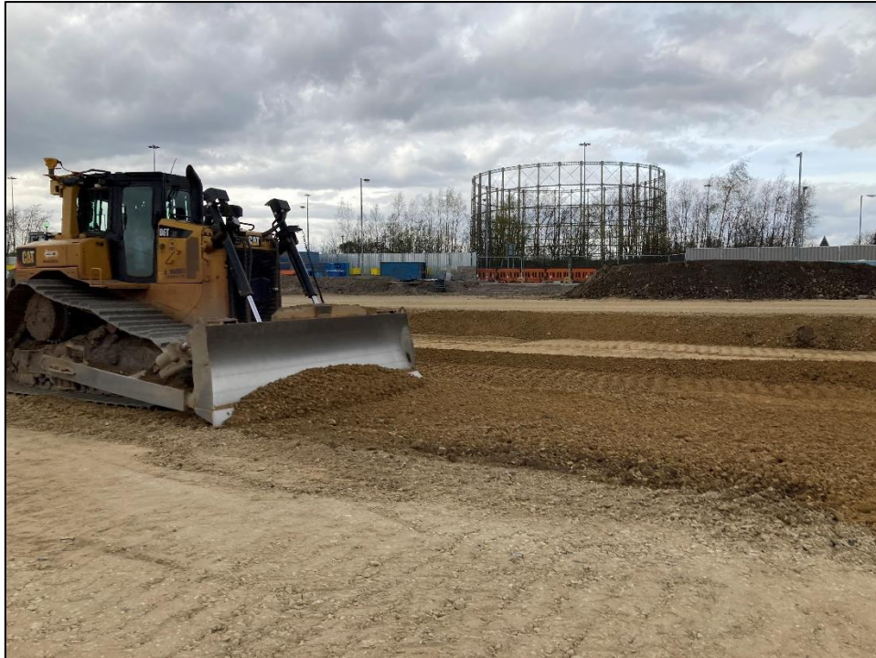
Photo 9 - Trimming of Pile Mat Levels
