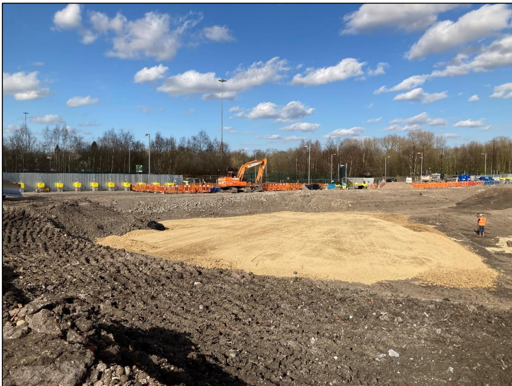
Photo 4 - Placement of Low Level Pile Mat
