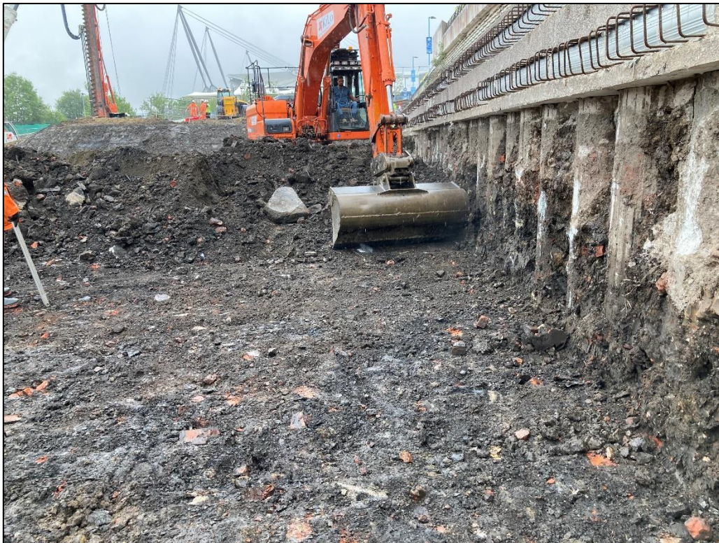
Photo 22 – Excavation to Formation
