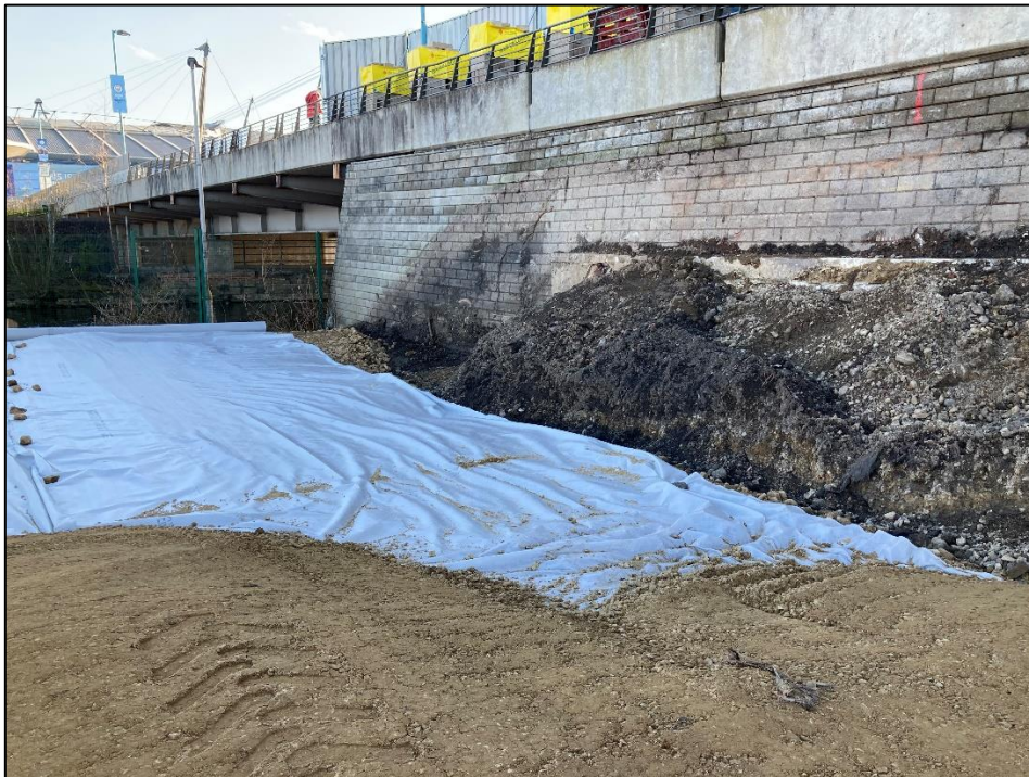
Photo 6 Placement of Upper Level Pile Mat
