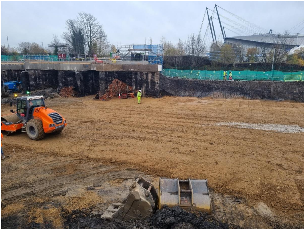
Photo 33 – Final Pile Mat Area on South of Site
