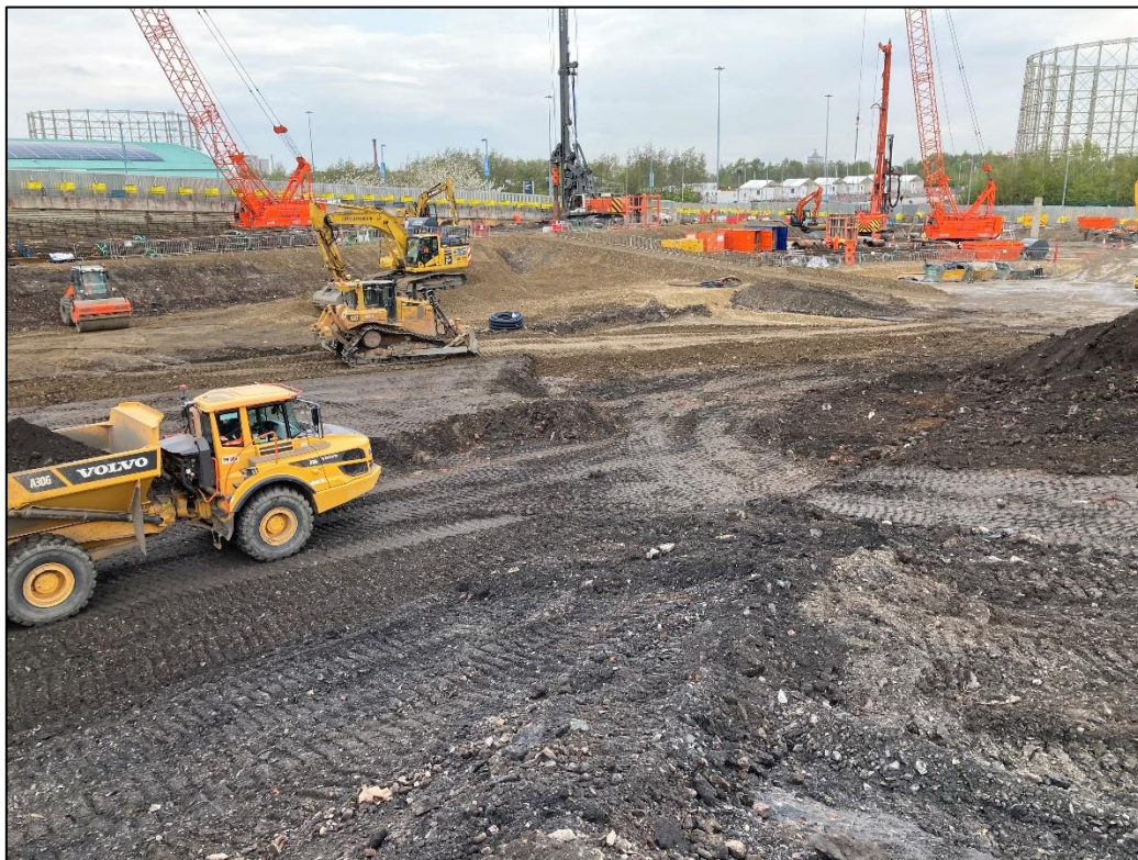
Photo 12 Low Level Mat Earthworks
