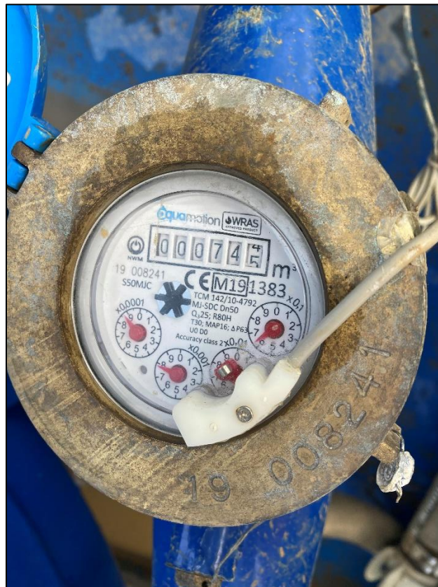
Photo 8 Flowmeter Reading for Groundwater Treatment System
