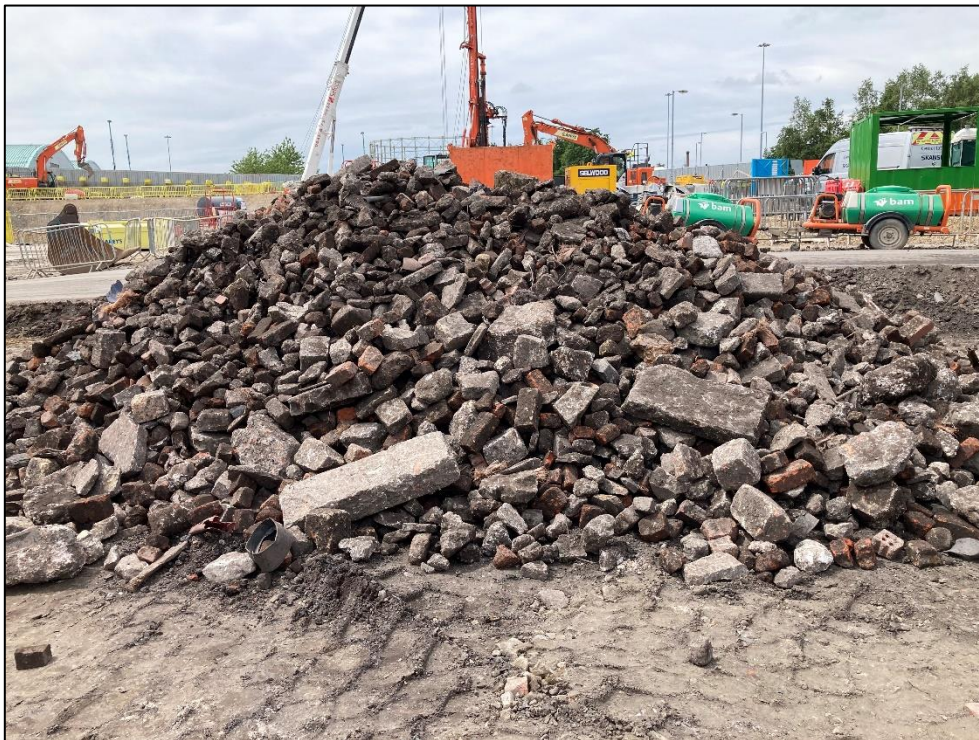
Photo 16 Stockpile of Concrete and Bricks
