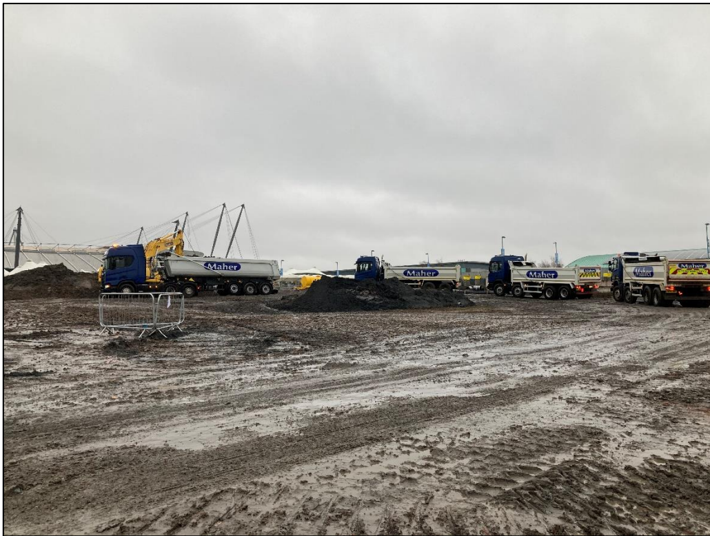
Photo 4 - Placement of Low Level Pile Mat
