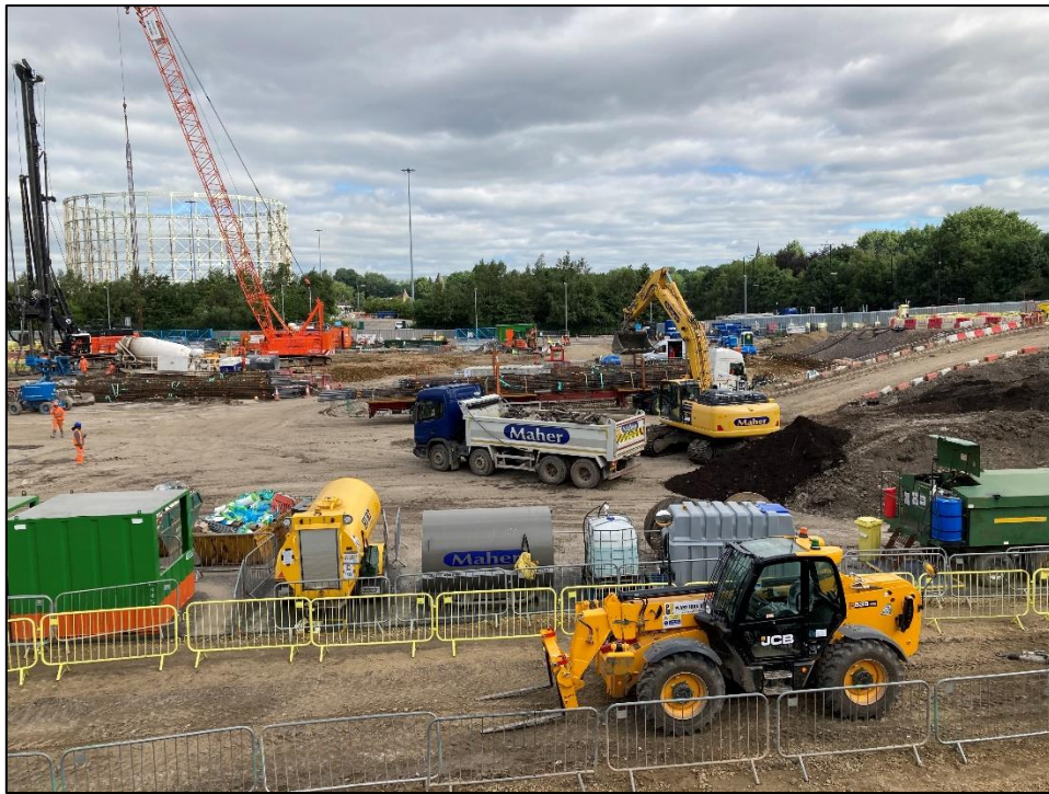
Photo 24 – Bulk Excavation of Material
