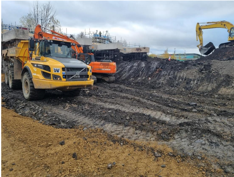
Photo 32 – Stockpiling and Muckaway Point
