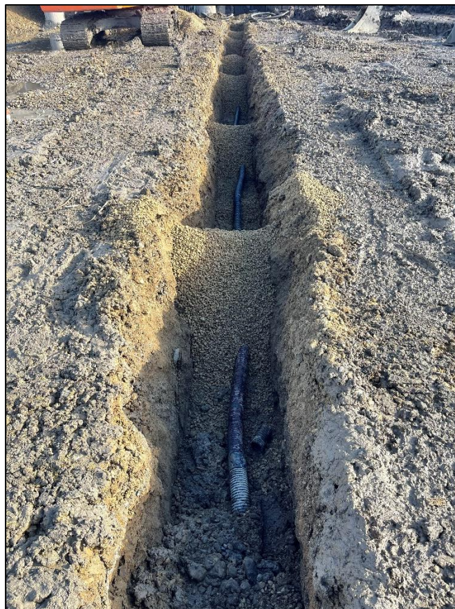
Photo 28 – Installation of Temporary Surface Water Drainage
