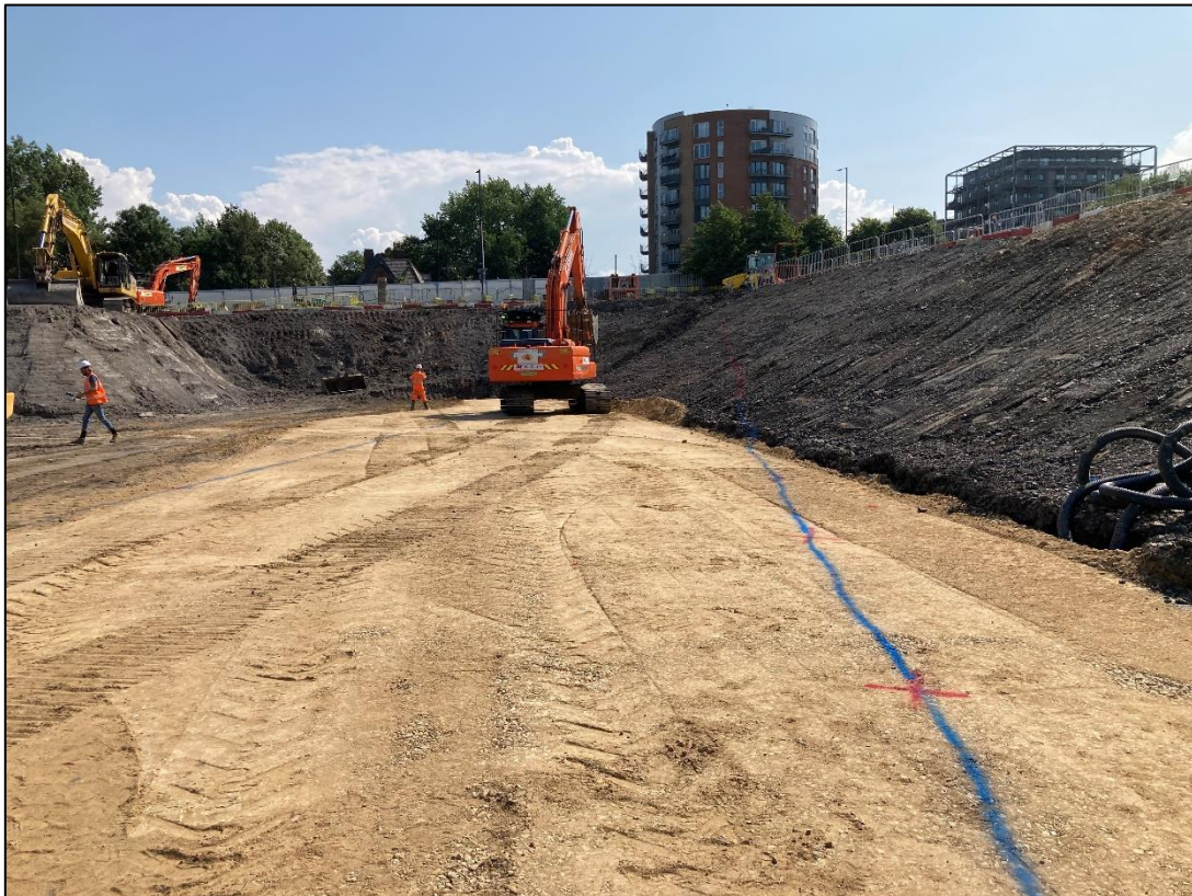
Photo 26 - Low Level Pile Mat in Central Bowl Area
