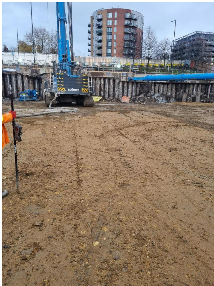
Photo 30 – Pile Mat in Southeast Corner of Site
