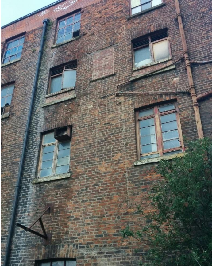
Figure 6 - Modern brickwork infill at second floor (taken 2018)
