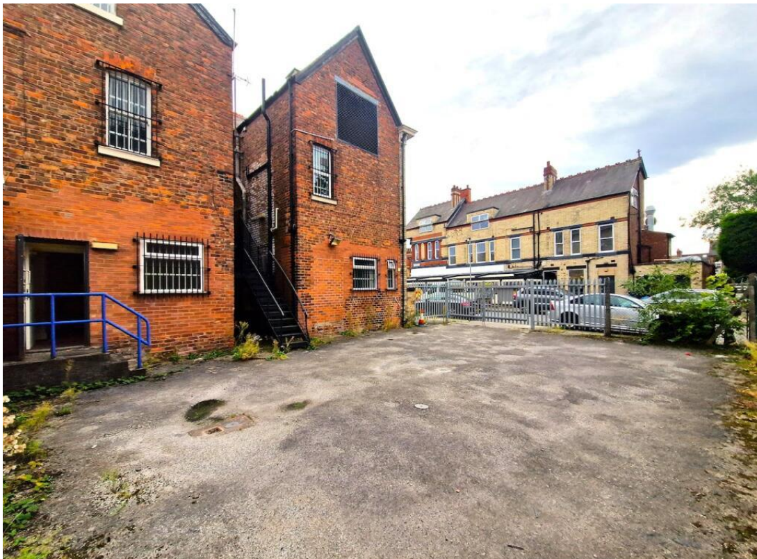
Image 3 – Photograph of rear elevation and car park facing towards Silverwood Avenue
