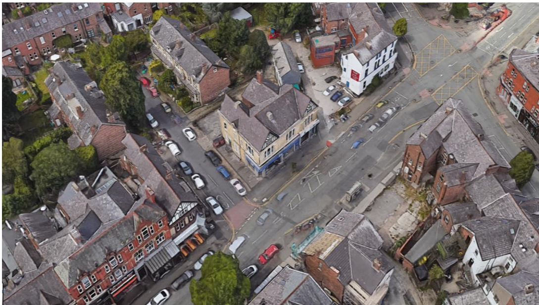
Image 5 – Overhead view of site facing north west
