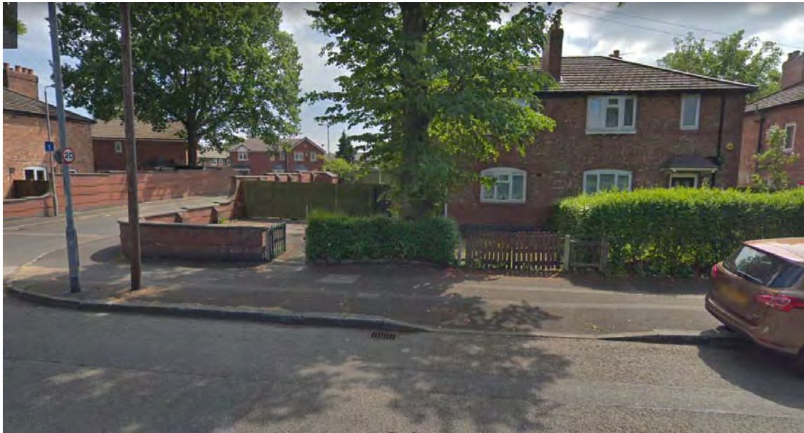
Figure 3.1: No.121 Mauldeth Road West, Withington
