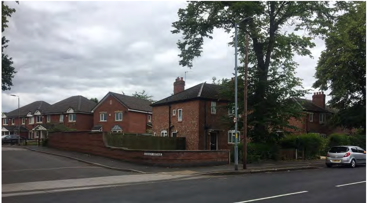
View to site from Mauldeth Road West
