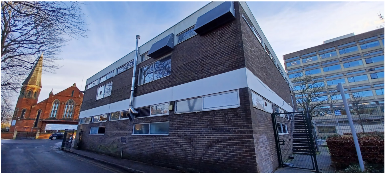
Figure 2. Elevation facing site access road.
