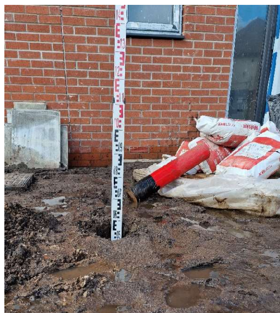
Depth of pit demonstrated at 600mm
