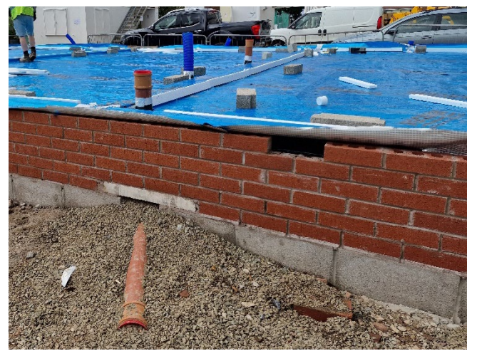
Figure 4 – Sufficient vents can be seen (every 2m).
