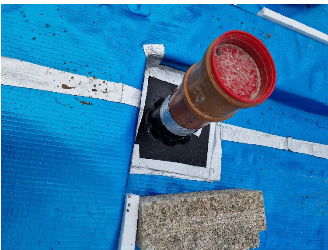
Figure 3 – Corners installed using detailing tape giving sufficient coverage of cavities
