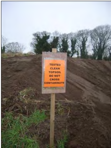
Photographs 7 & 8: Example of good stockpile management with warning signs to demonstrate areas of inert topsoil
