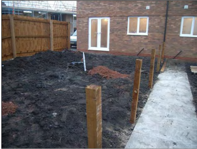
Photographs 2 & 3: Examples of validation photographs demonstrating inert cover
