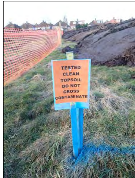
Photographs 7 & 8: Example of good stockpile management with warning signs to demonstrate areas of inert topsoil
