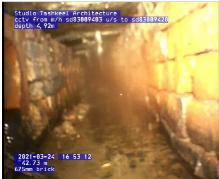
Photo: 1_1_35_A.jpg 42.73m, Connection other than junction, at 9 o'clock, diameter 225mm
