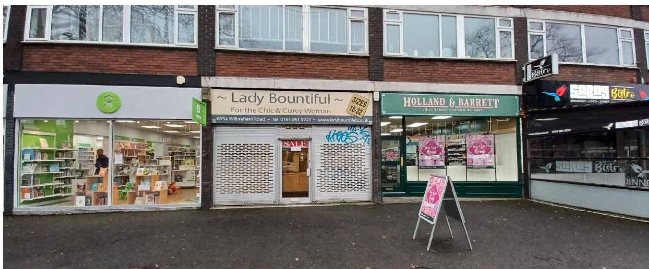
Figure 1. Photograph of the principal elevation of No.605A Wilbraham Road.
