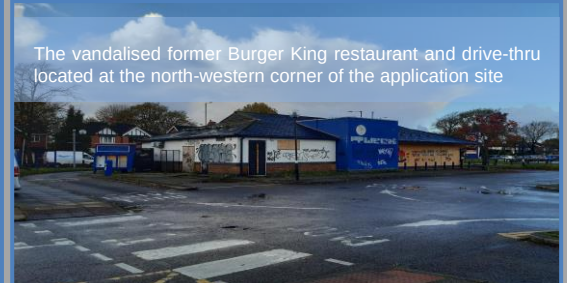
The commercial units north of the application site at the northern end of the Fallowfield Retail Park
