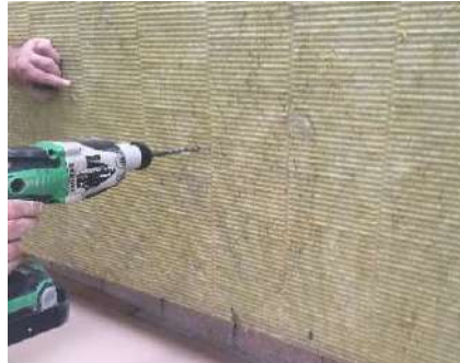
Preparation of wall & Installation of insulation
