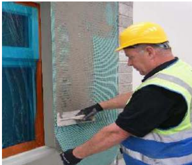
Preparation of wall & Installation of insulation
