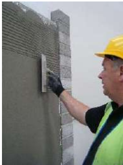
Installation of substrate
