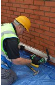
Preparation of wall & Installation of insulation
