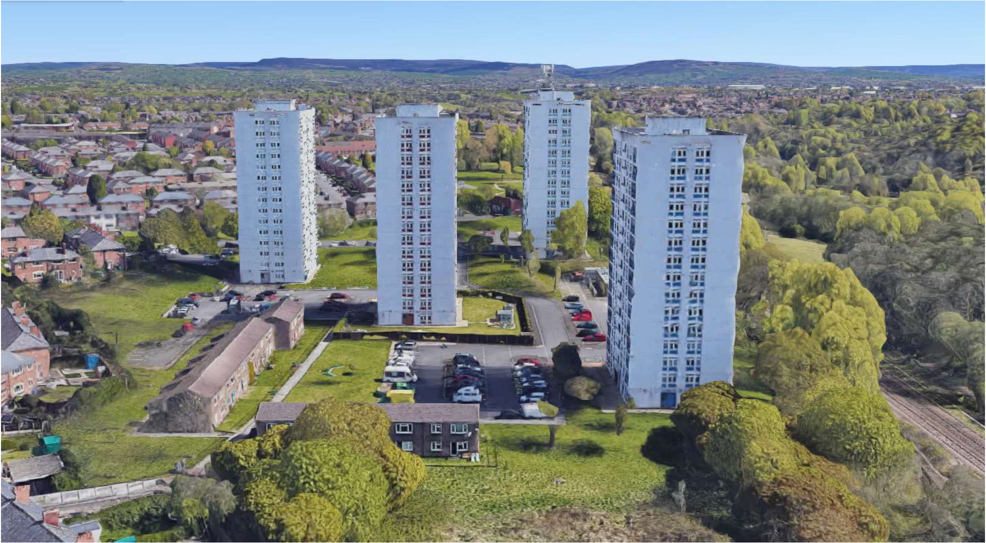
Avro Hollows site (looking east). Low-rise blocks: Audax Walk (left), Underhill Walk (Centre) High-rise blocks (from left to right): Lancaster Court, Dobson Court, Shackleton Court, Lincoln Court
