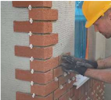
Application of brick slips
