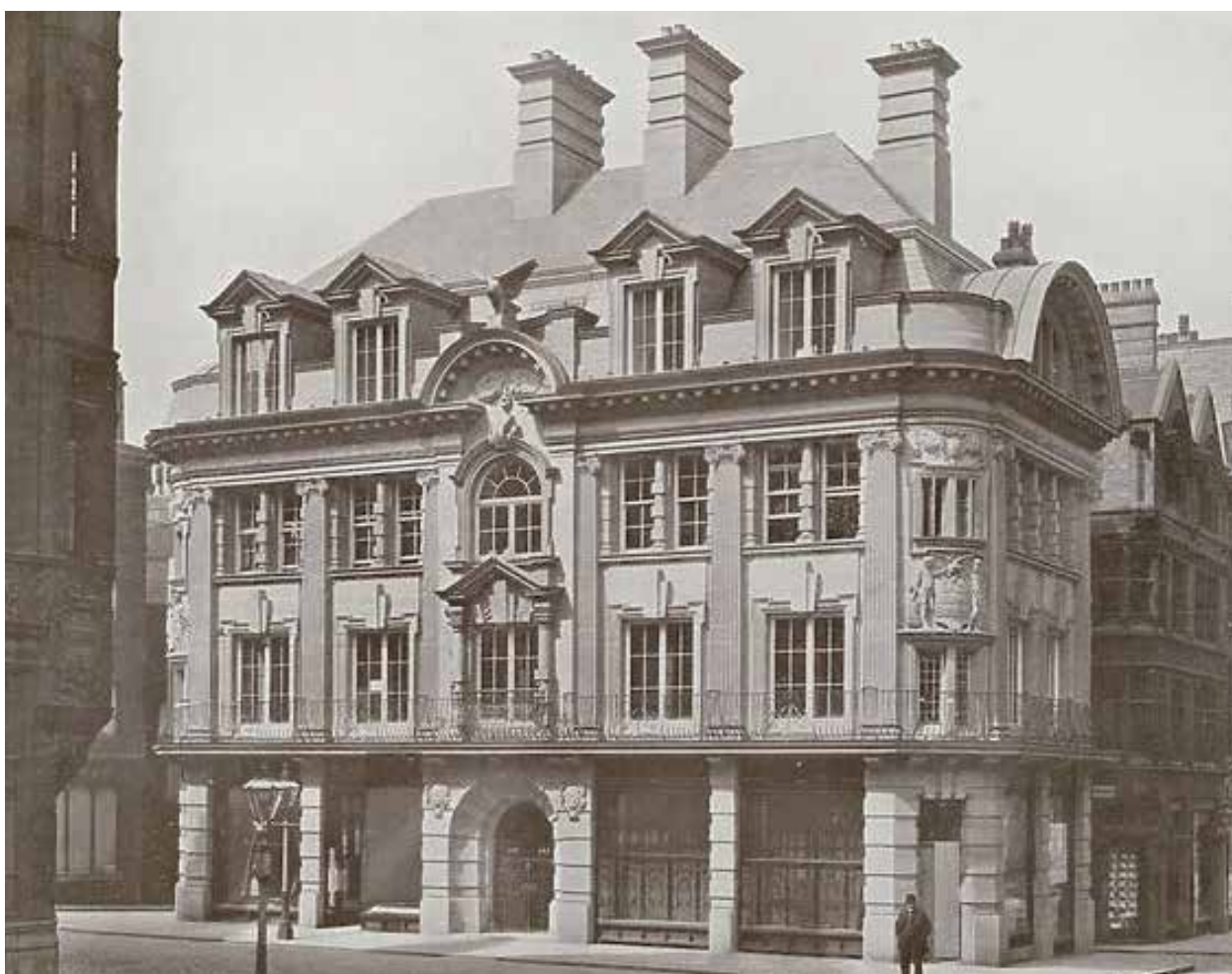
Figure 2.2 A photograph of the Eagle Insurance Co's Office, Manchester (unknown date)
