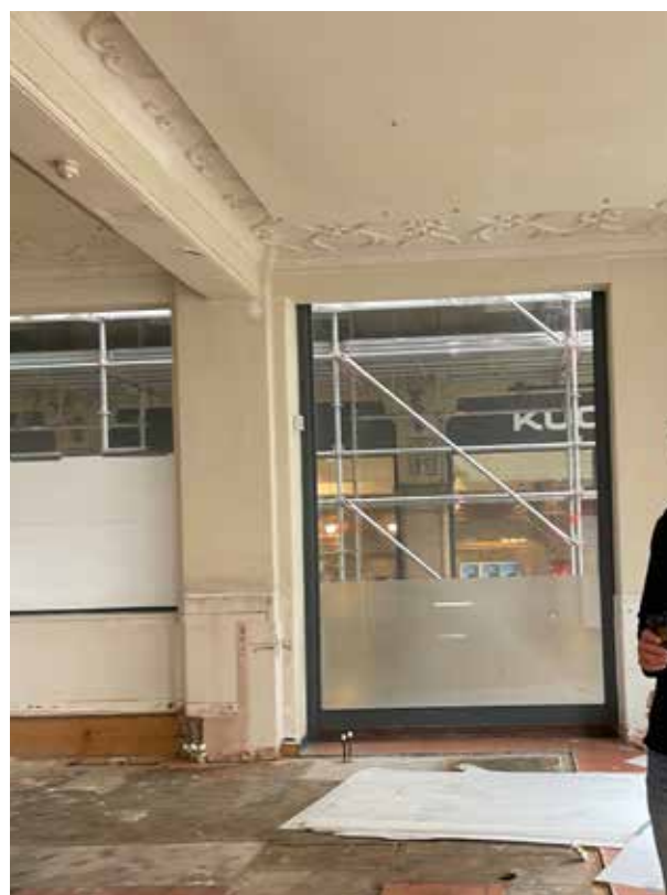
Figure 4.22 Ground floor: modern frosting vinyl to be removed from window.
