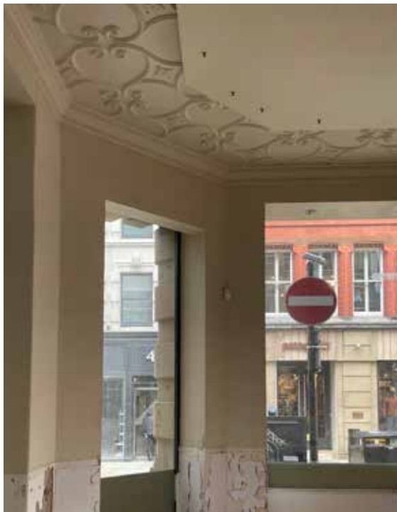
Figure 2.11 Site photograph showing decorative ceiling detailing on ground floor.
