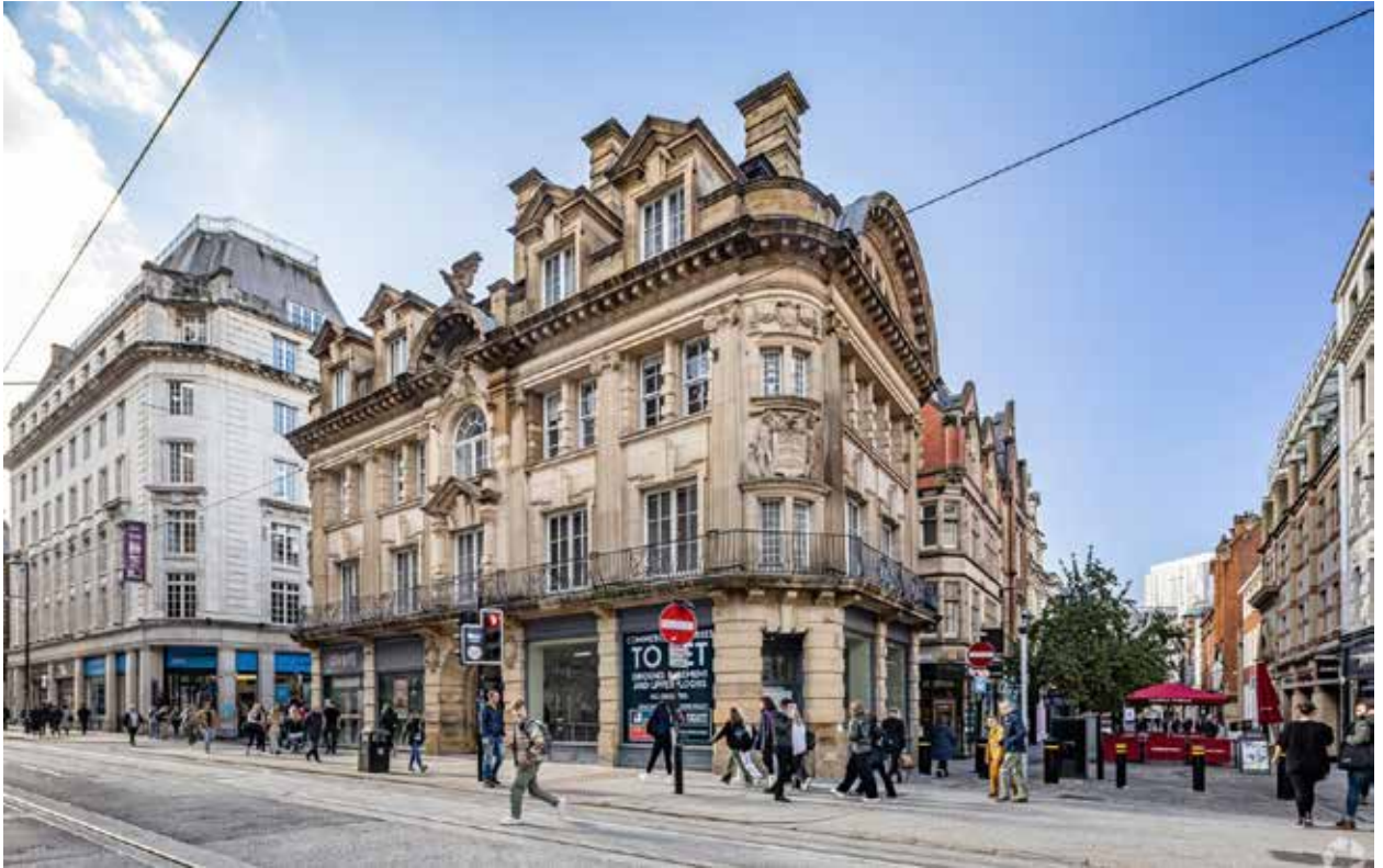
Figure 2.6 Photograph showing the site as it currently is, an empty commercial premises.
