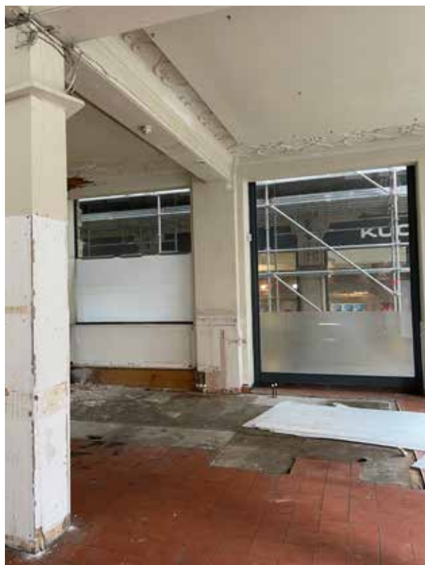
Figure 4.16 Ground floor: modern ceiling panels attached to historic decorative ceiling. Existing panels to be repurposed for lighting to minimise damage to historic ceiling.
