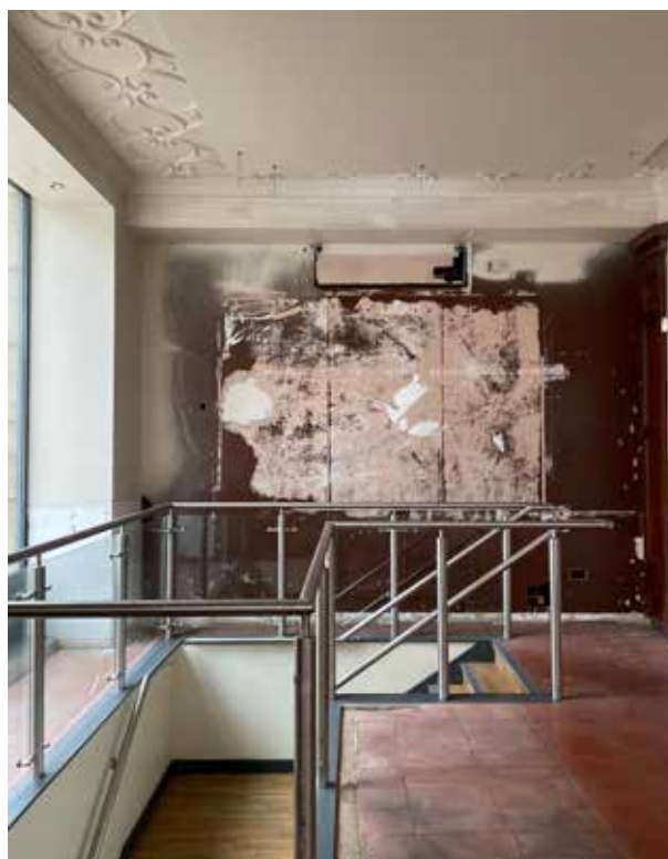
Figure 4.18 Ground floor: Modern plasterboard to be removed to expose existing plasterwork or original brick work.
