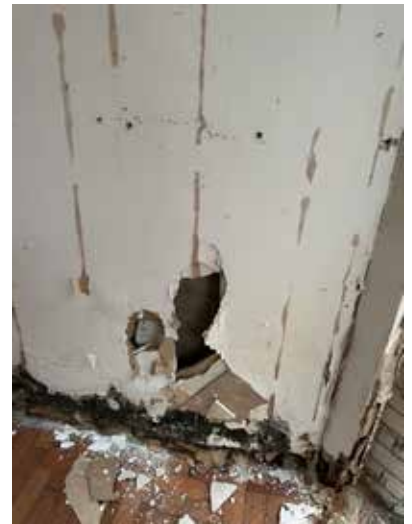
Figure 4.9 & 4.10 Basement: modern plasterboard structure (with damp membrane behind) and wall finish to be repaired and made good.
