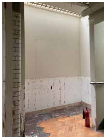
Figure 4.11 Basement: existing Altro flooring to be replaced as intend to use for dried food & storage. Existing parquet flooring retained.
