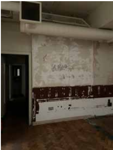
Figure 4.8 Basement: modern plasterboard and wall finish to be repaired and made good to match existing.
