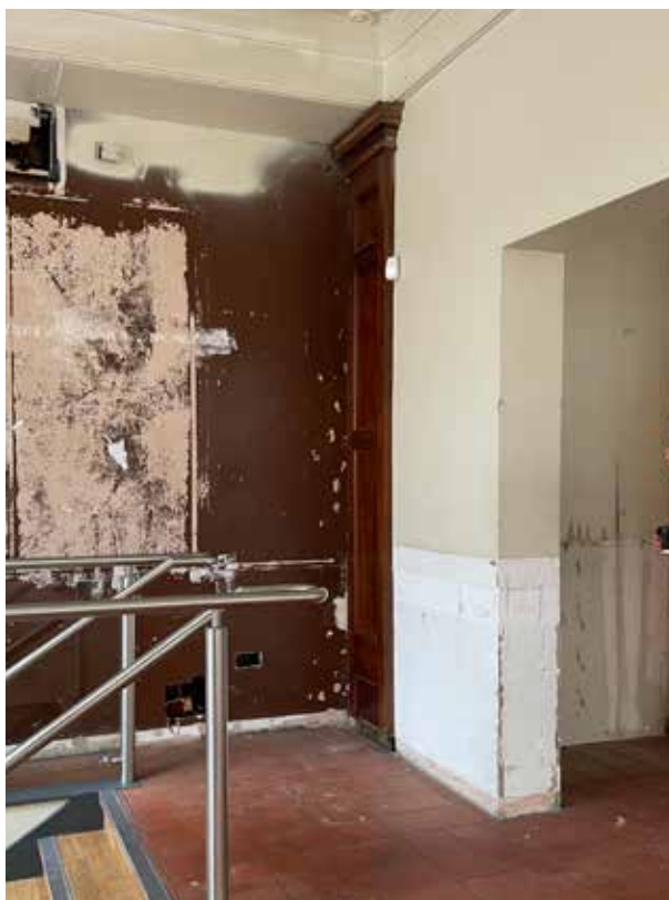
Figure 4.19 Ground floor: modern stained plywood feature to be removed. Works will not comprise the historic ceiling and the modern panels.
