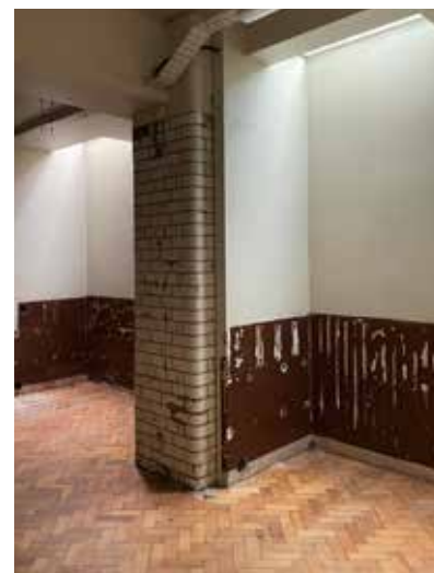
Figure 4.13 Basement: ceiling to be redecorated. New heads to be affixed to fire system. Lighting to be installed on either existing tray work or areas where lighting has been removed. All fresh air ducting to remain and serviced only.
