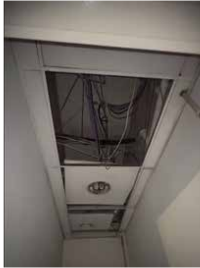
Figure 4.6 Basement: existing suspended ceiling and services to bathrooms.
