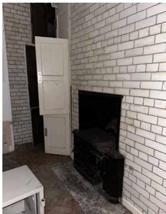
Figure 2.8 Site photograph within basement of one of the cast iron fireplaces surrounded by glazed brickwork
