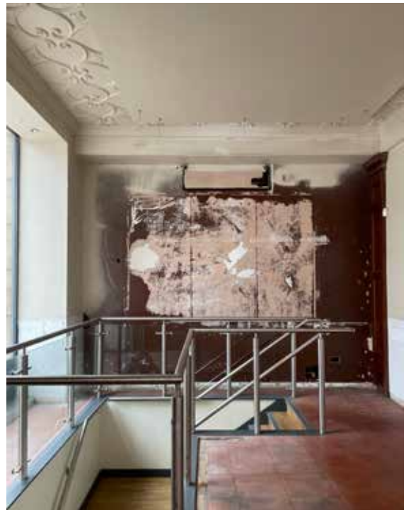
Figure 2.12 Site photograph of ground floor showing existing staircase balustrade to basement and decorative ceiling detailing.
