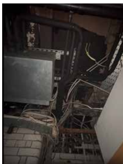
Figure 4.2 Basement: existing services to ceiling in room with fire place along rear elevation (Fourth Yard).
