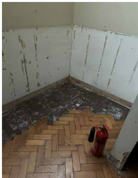
Figure 2.10 Site photograph within basement of original parquet flooring
