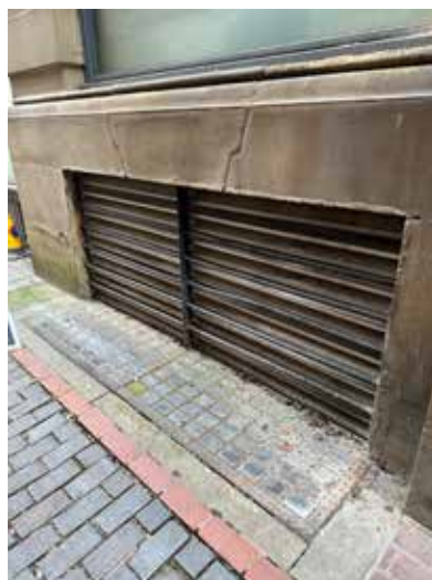
Figure 4.12 Existing louvres on Four Yards elevation.
