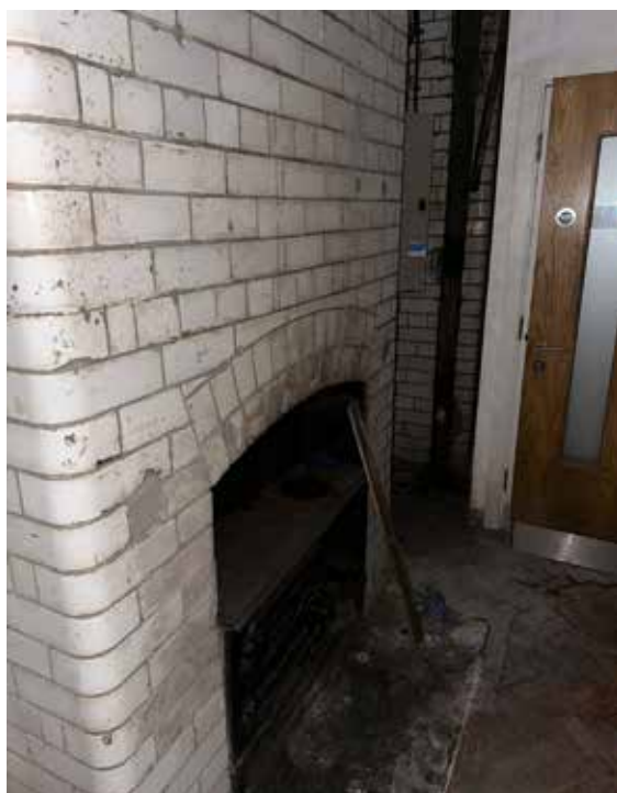
Figure 2.9 Site photograph within basement of one of the cast iron fireplaces surrounded by glazed brickwork
