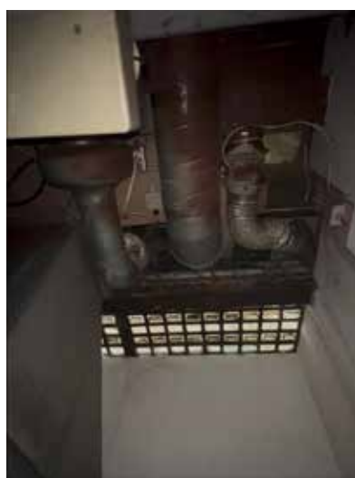
Figure 4.3 Basement: existing services to louvres riser along Fourth Yard elevation.
