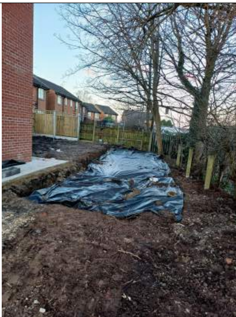
Photograph 2: Validation of membrane placement
