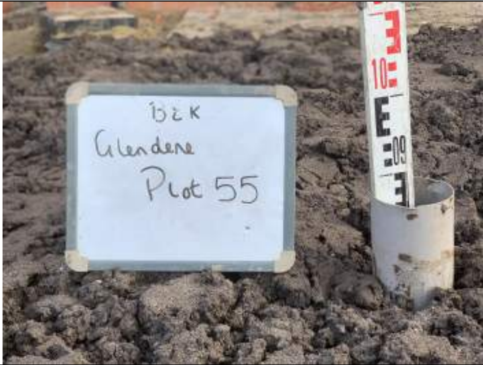
Photograph 1: Validation of Garden Capping
