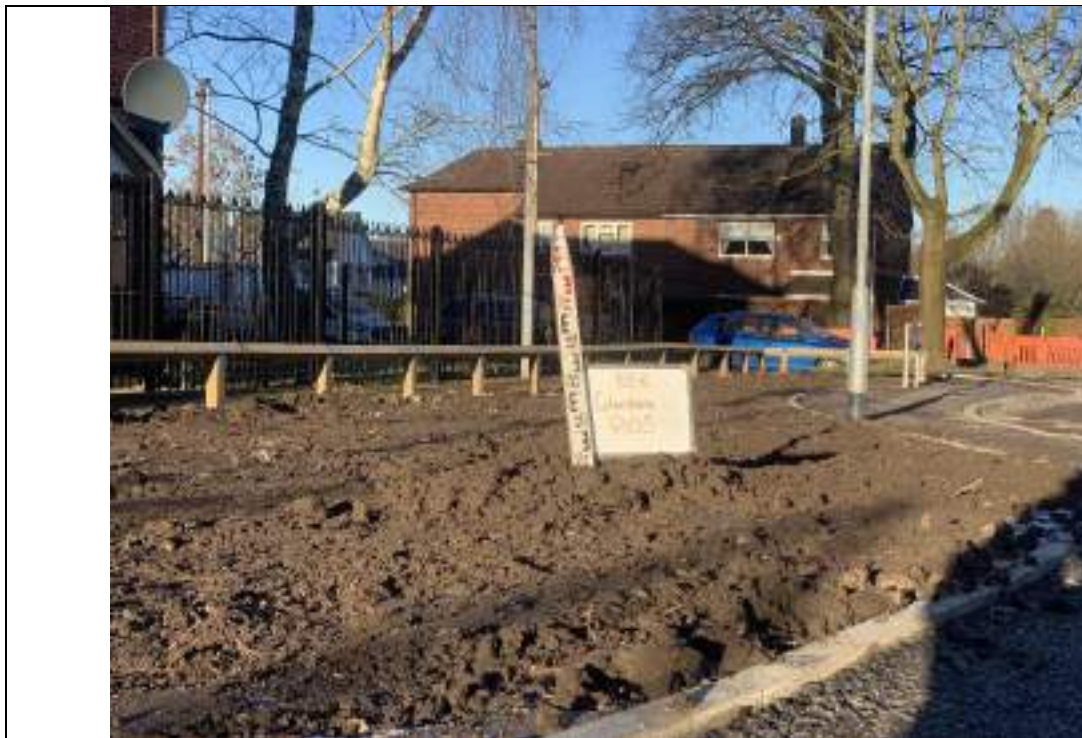
Photograph 2: Validation of Public Open Space Capping
