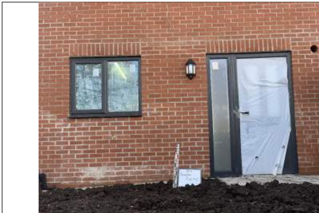
Photograph 2: Validation of Garden Capping
