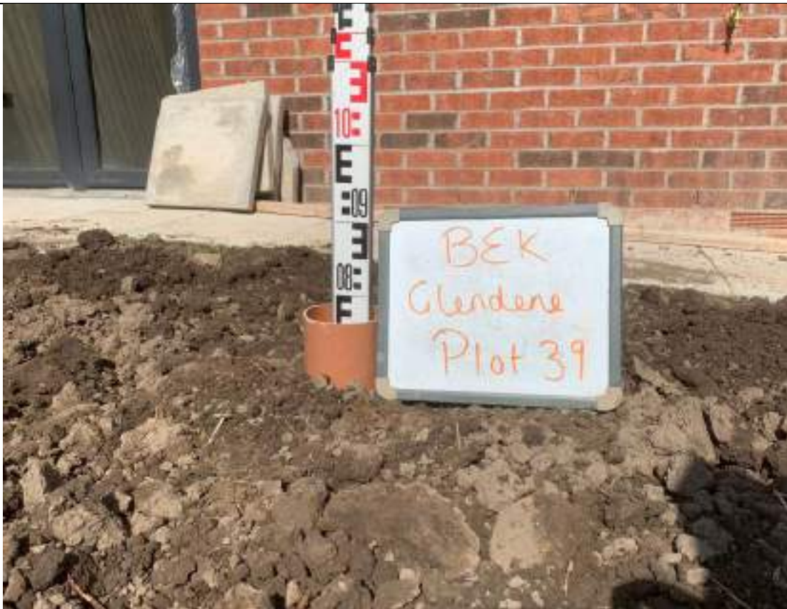
Photograph 1: Validation of Garden Capping
