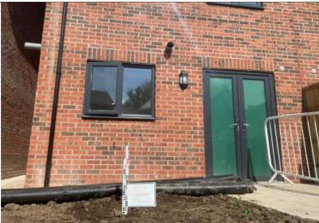
Photograph 2: Validation of Garden Capping
