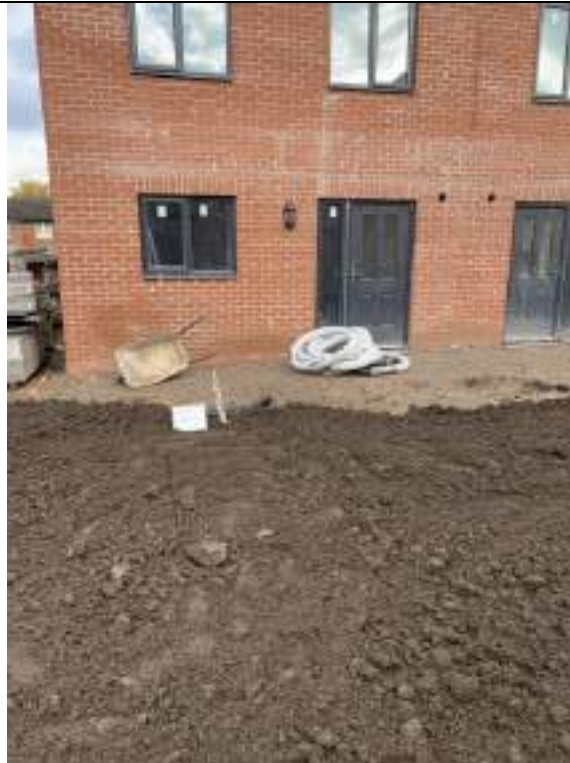
Photograph 2: Validation of Garden Capping
