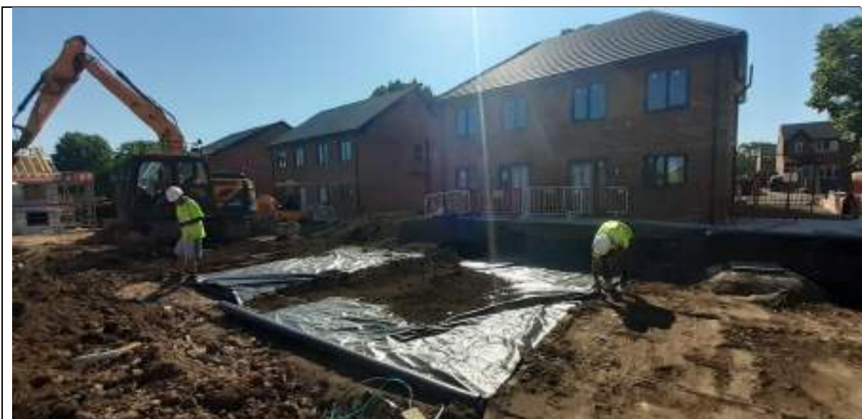
Photograph 1: Validation of membrane placement
