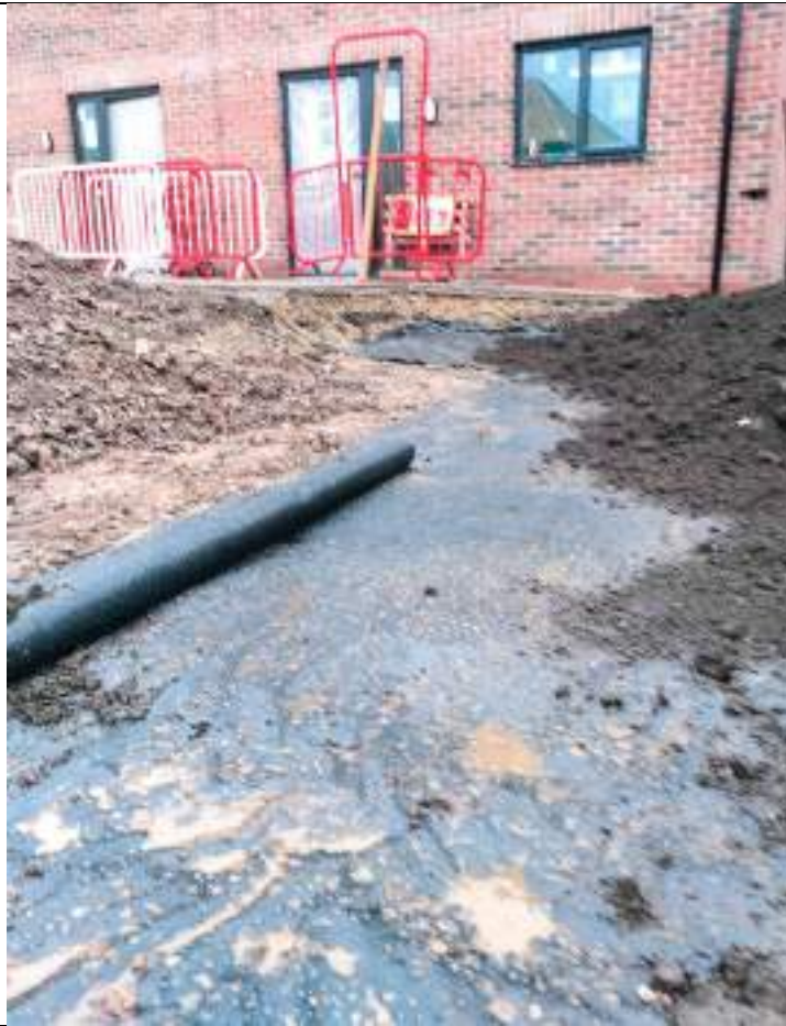
Photograph 5: Validation of membrane placement in Plot 21
