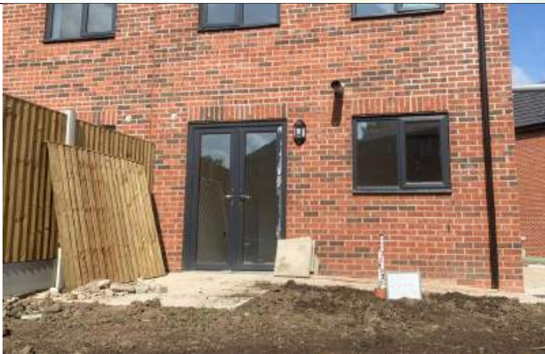
Photograph 2: Validation of Garden Capping
