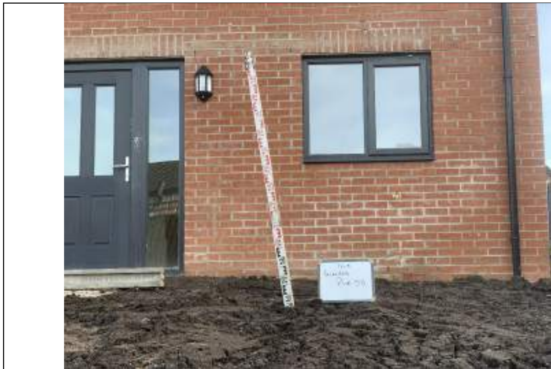
Photograph 2: Validation of Garden Capping
