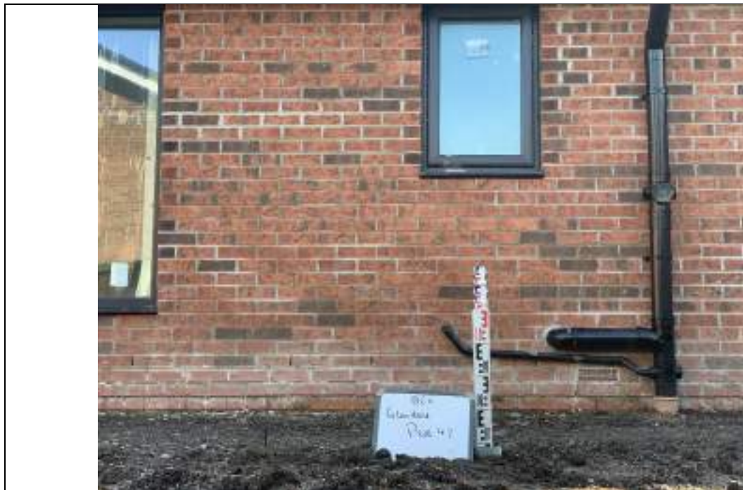
Photograph 2: Validation of Garden Capping
