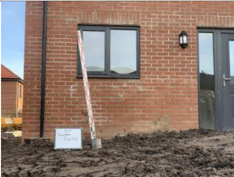
Photograph 2: Validation of Garden Capping
