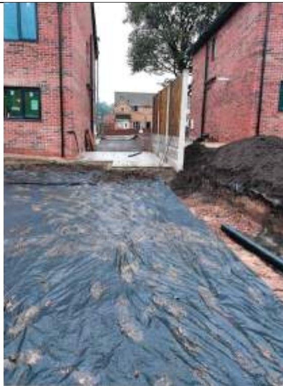
Photograph 6: Validation of membrane placement in Plot 20
