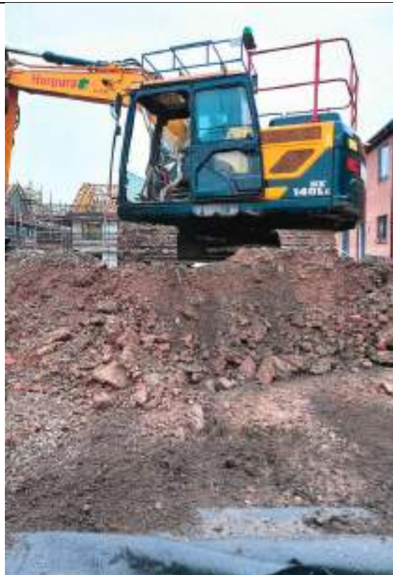
Photograph 4: Validation of membrane placement in Plot 20
