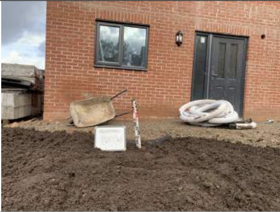
Photograph 1: Validation of Garden Capping
