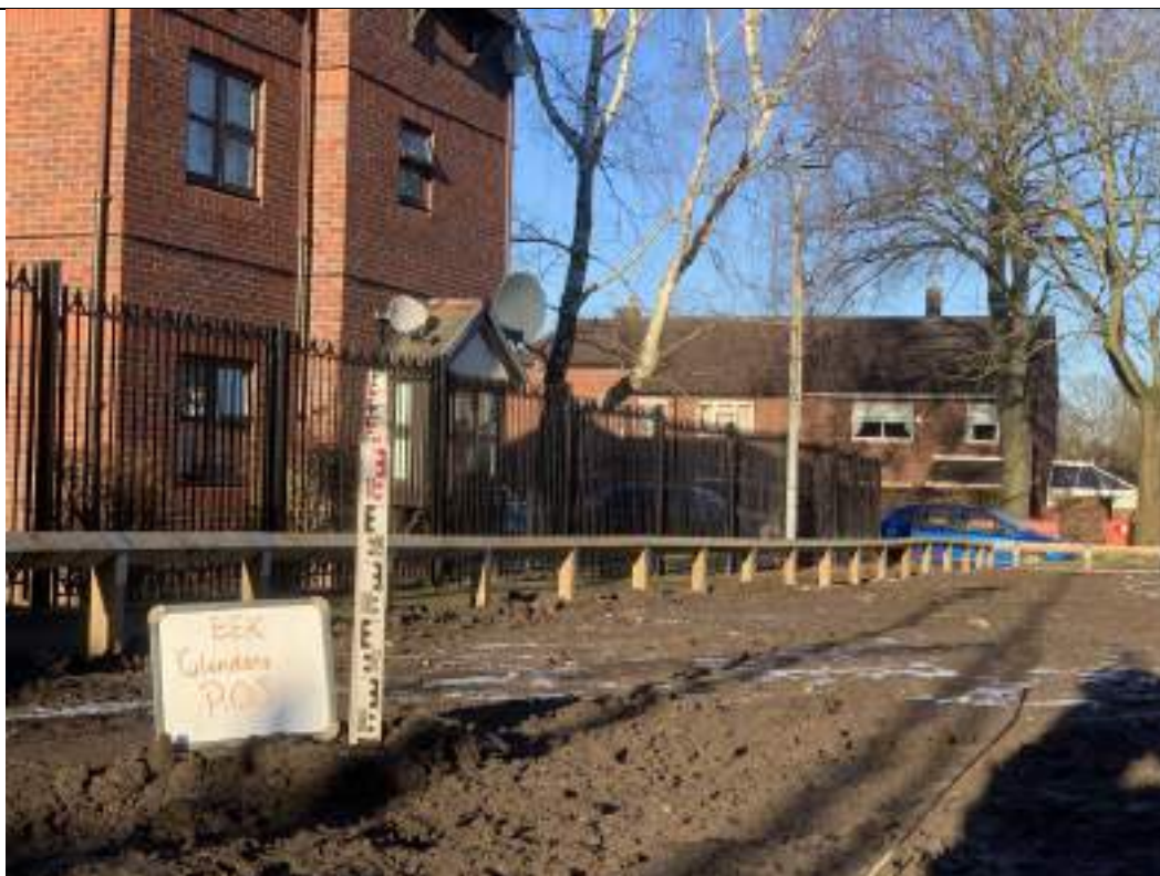
Photograph 4: Validation of Public Open Space Capping
