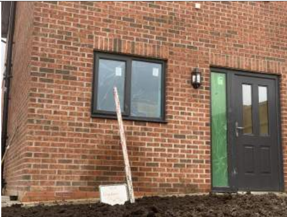
Photograph 2: Validation of Garden Capping
