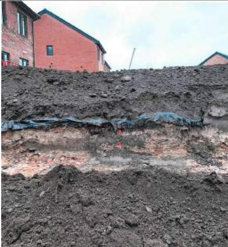
Photograph 3: Validation of membrane placement in Plot 16
