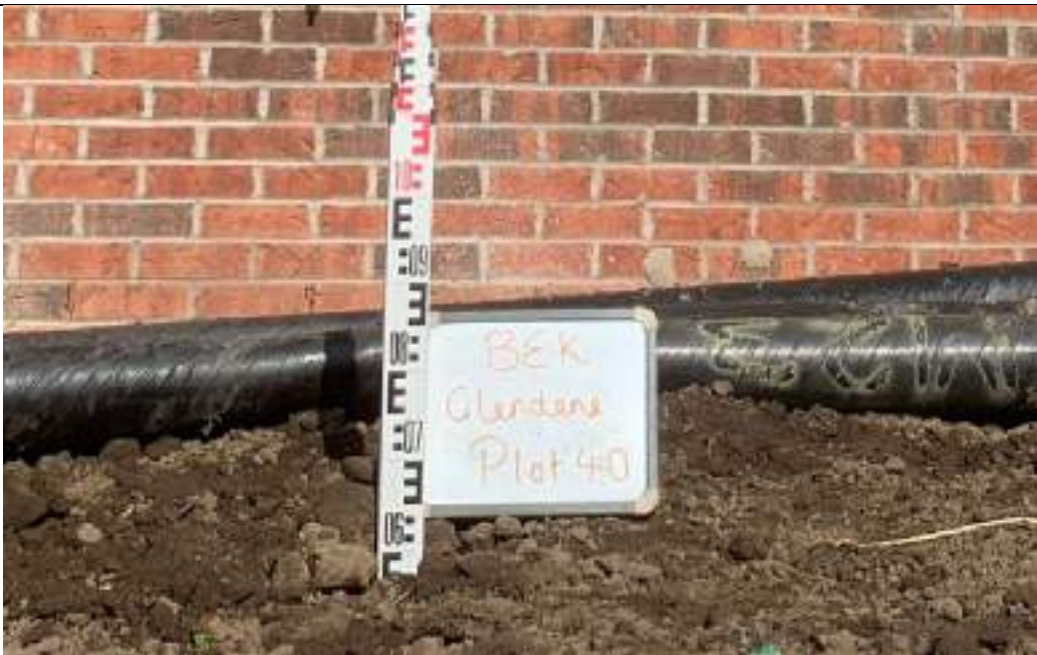
Photograph 1: Validation of Garden Capping
