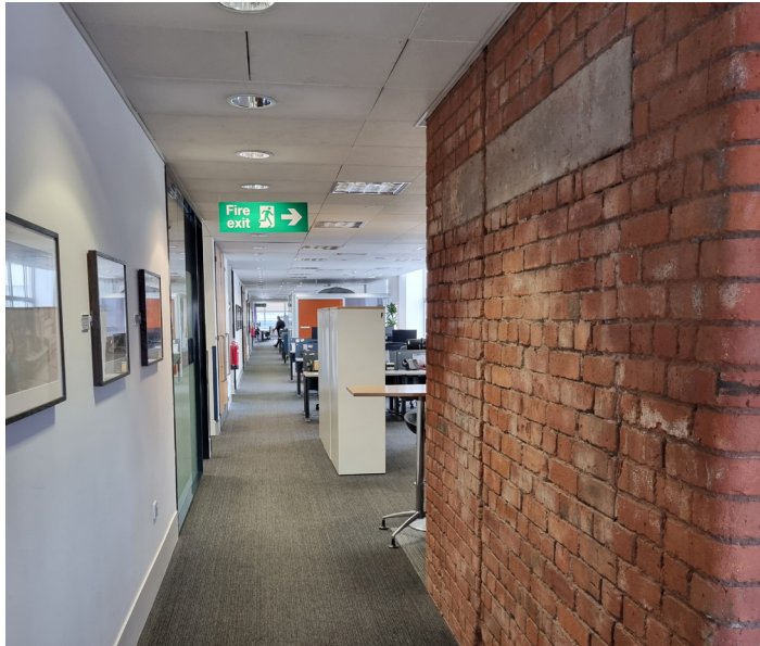
Rear of original brick shaft
