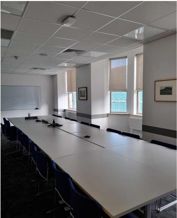
Windows to front elevation in meeting room
