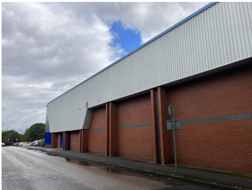
PLATE 1 SHOWING HARDSTANDING AND BUILDING
