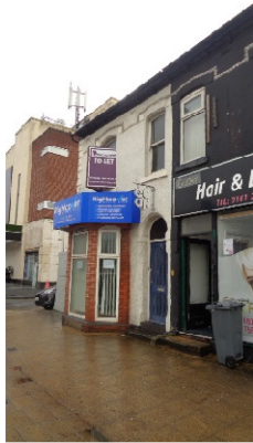
Front Elevation to Application Property.
