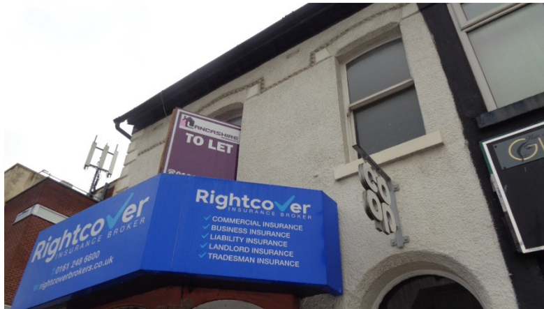
Front Elevation of Application Property.
